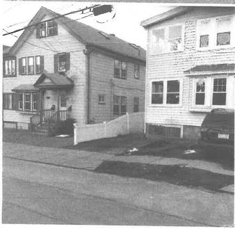
A tree had to be removed several years ago in front of our home 36-38 Upland. The roots had caused the sidewalk to rise and buckle as you can still see in the picture. The tree was removed but the sidewalk was not repaired.
