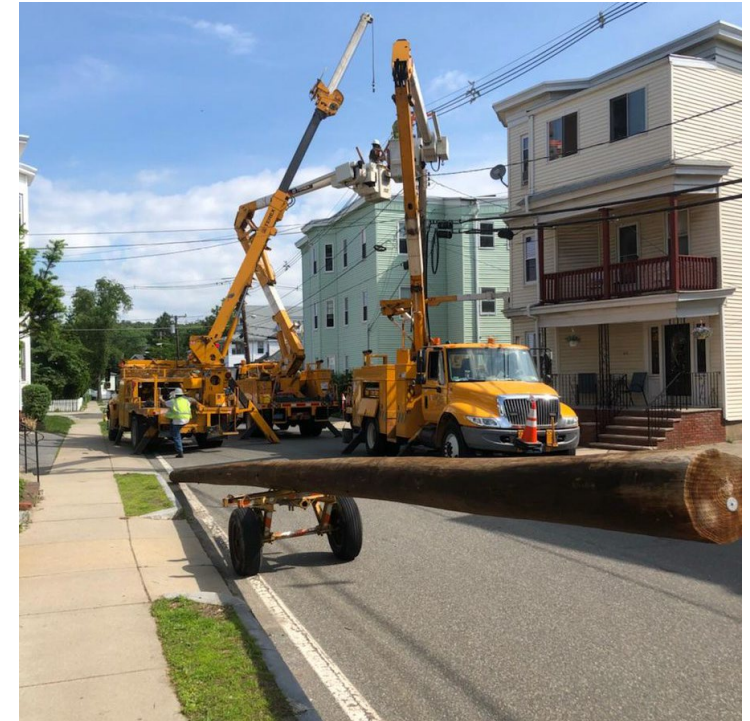
Photo: Routine pole and transformer replacement on Beech Street. Photo by Belmont Light, 2018, via Twitter.
