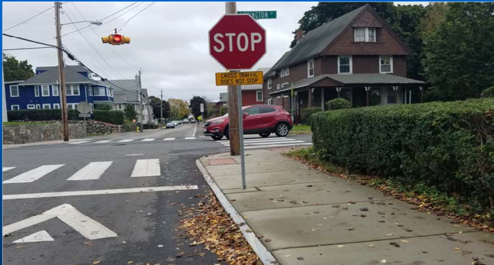
Sightline diminished by hedge at Sycamore Street eastbound approach
