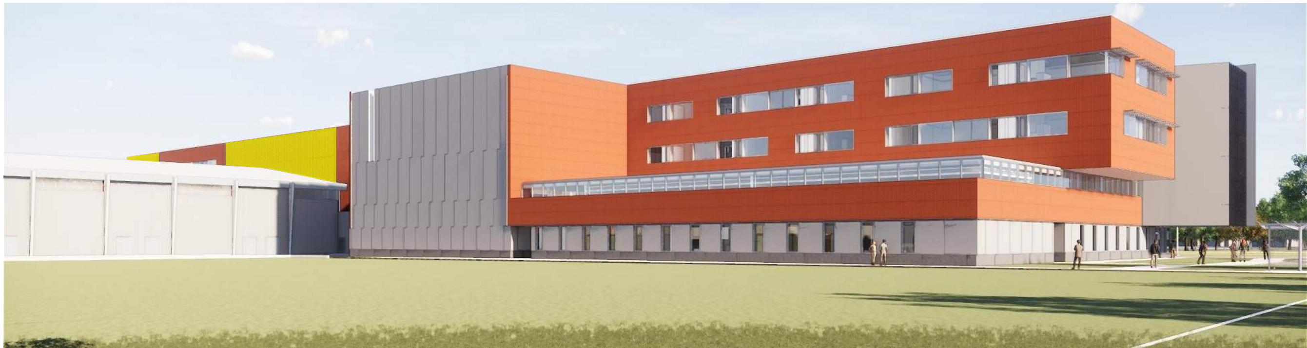
HIGH SCHOOL - BACK VIEW
