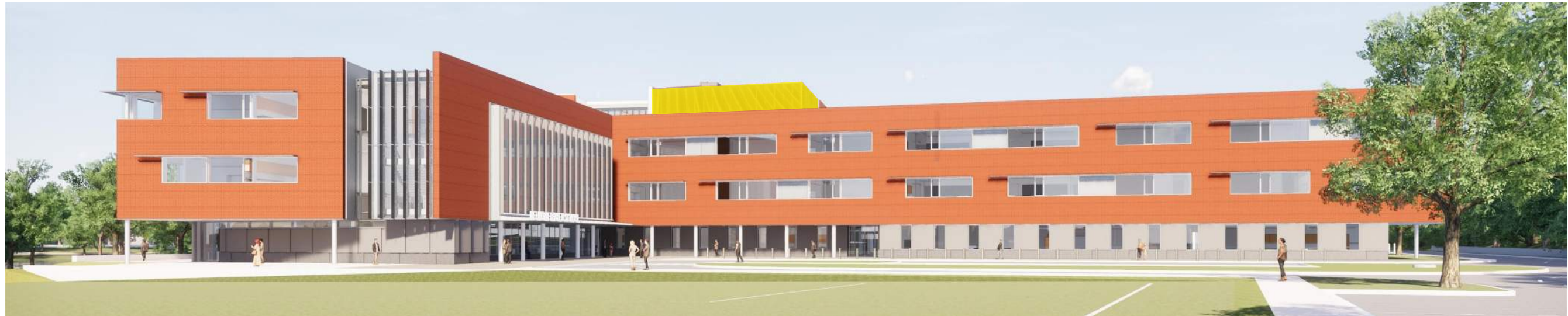
MIDDLE SCHOOL ENTRANCE
