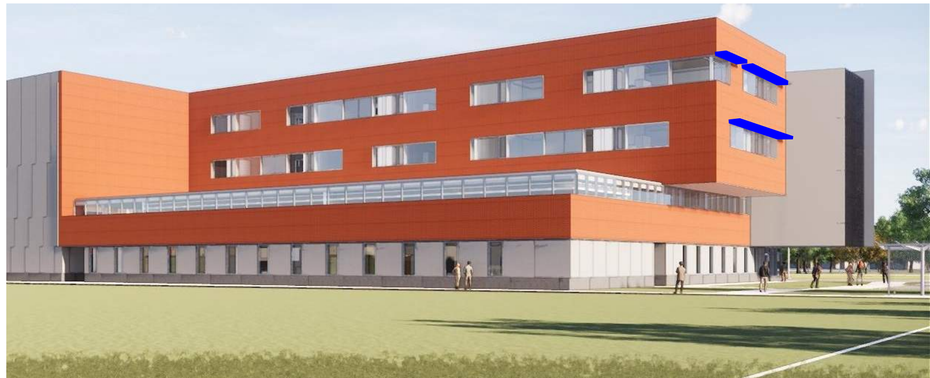
HIGH SCHOOL - BACK VIEW
