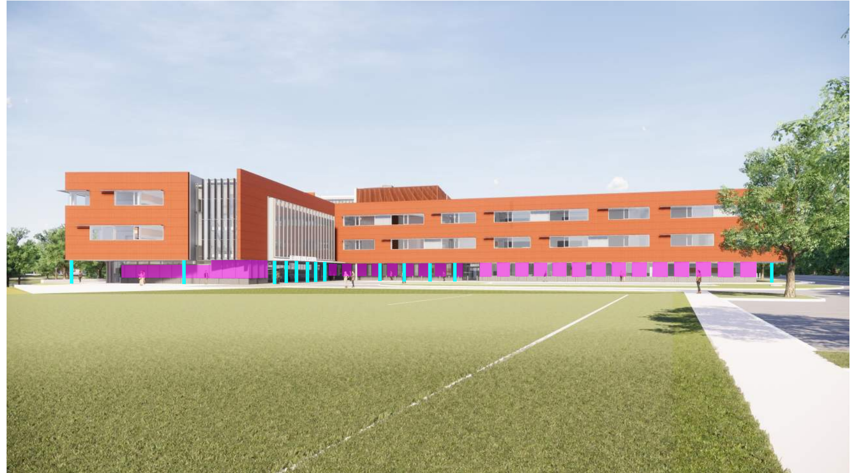
MIDDLE SCHOOL ENTRANCE
