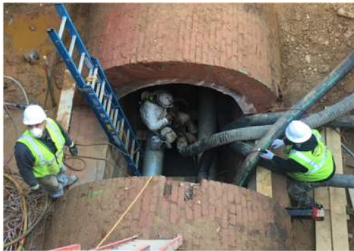
8' X 8' – EXISTING SEWER
