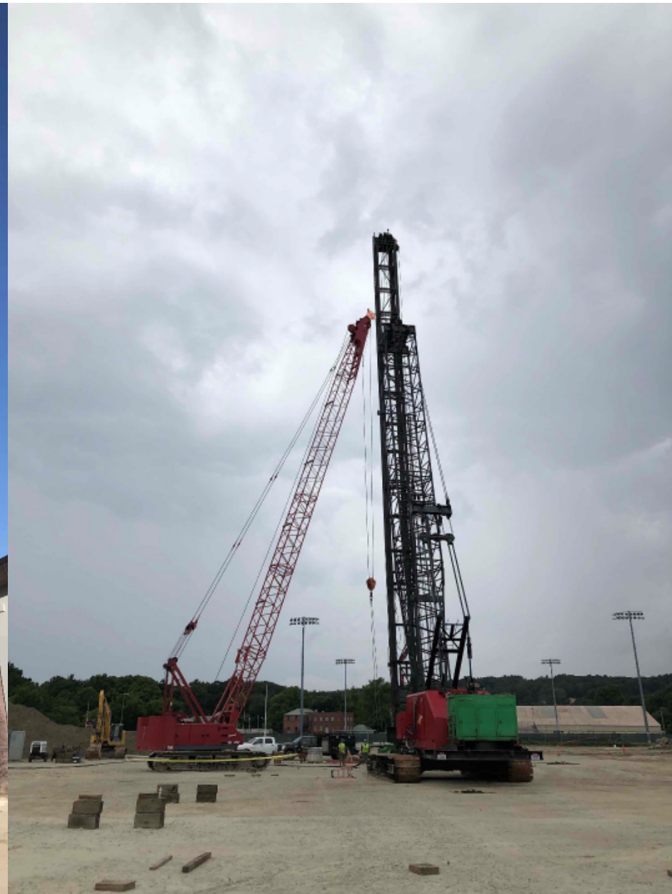
Photo 7 – Installation of Pile's for Foundation Elements.
