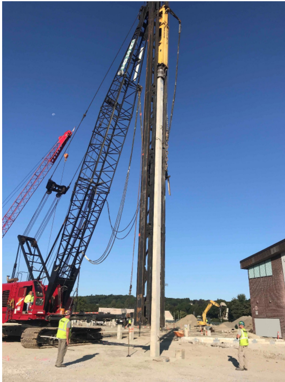
Photo 6 – Installation of Pile's for Foundation Elements.
