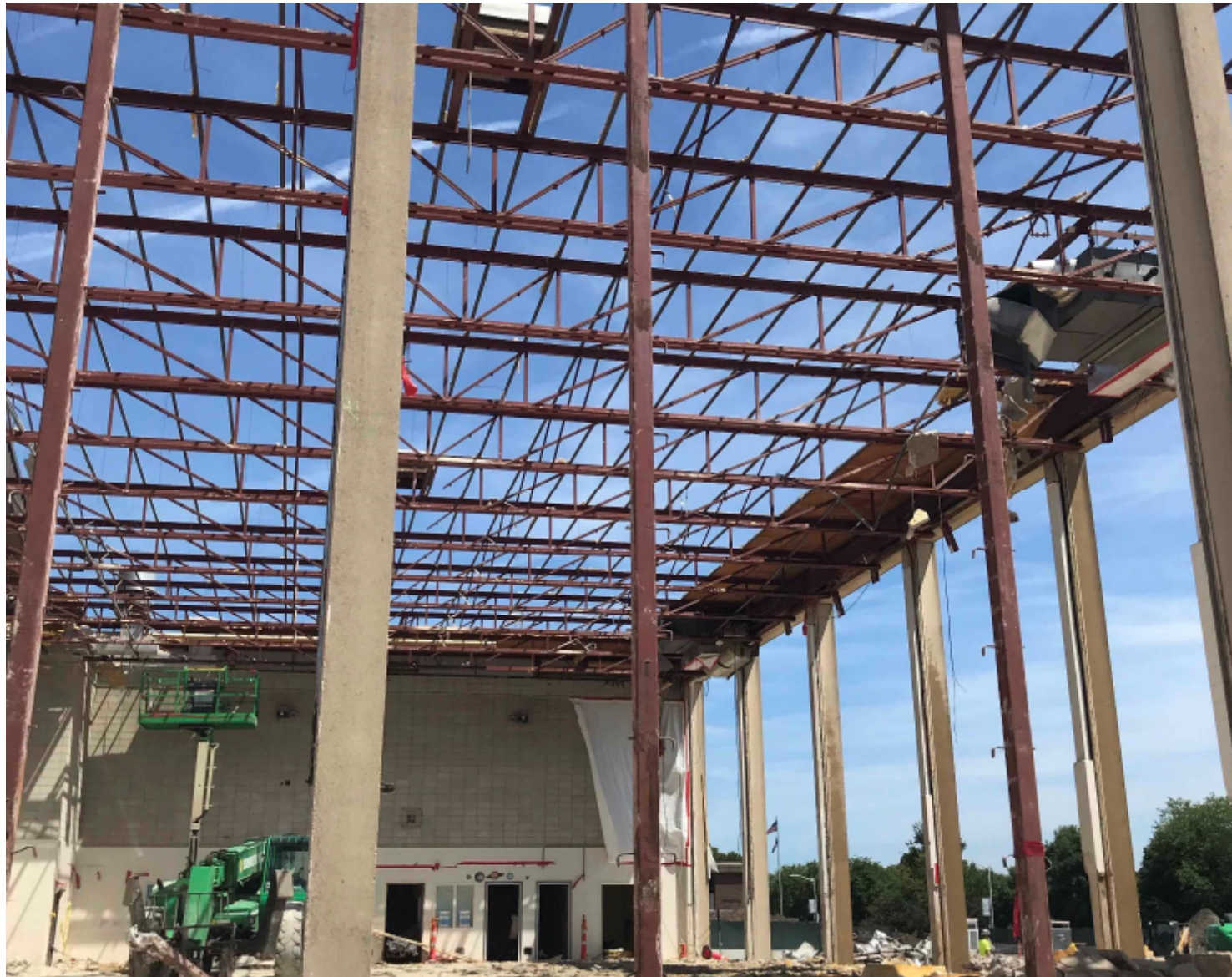
Photo 1 – Demolition Progress of Pool Structure.
