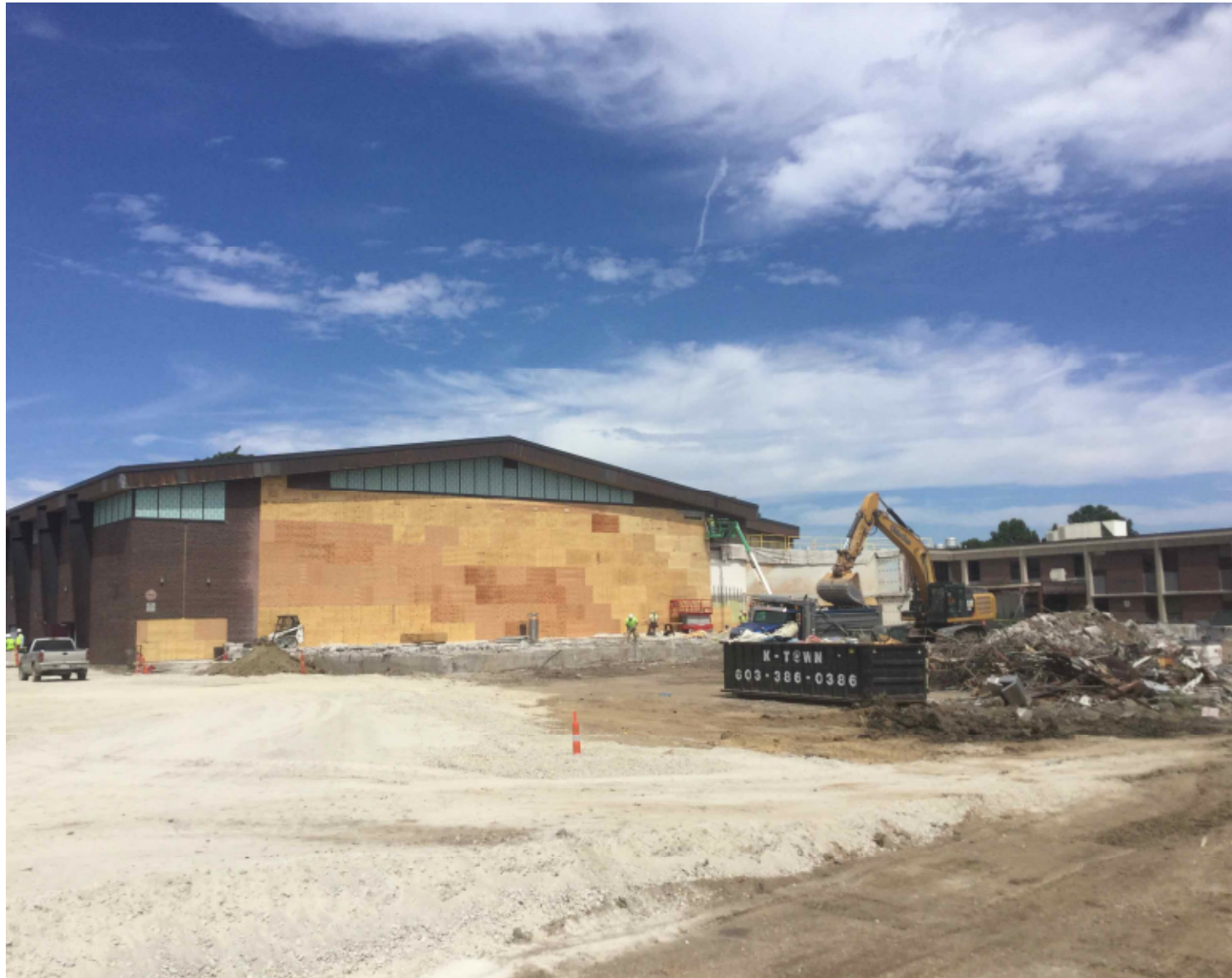
Photo 3 – Completion of Demolition and Installation of Field House Weather Barrier Plywood.
