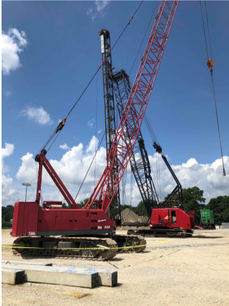
Photo 4 - Mobilization of Pile Driving Equipment.
