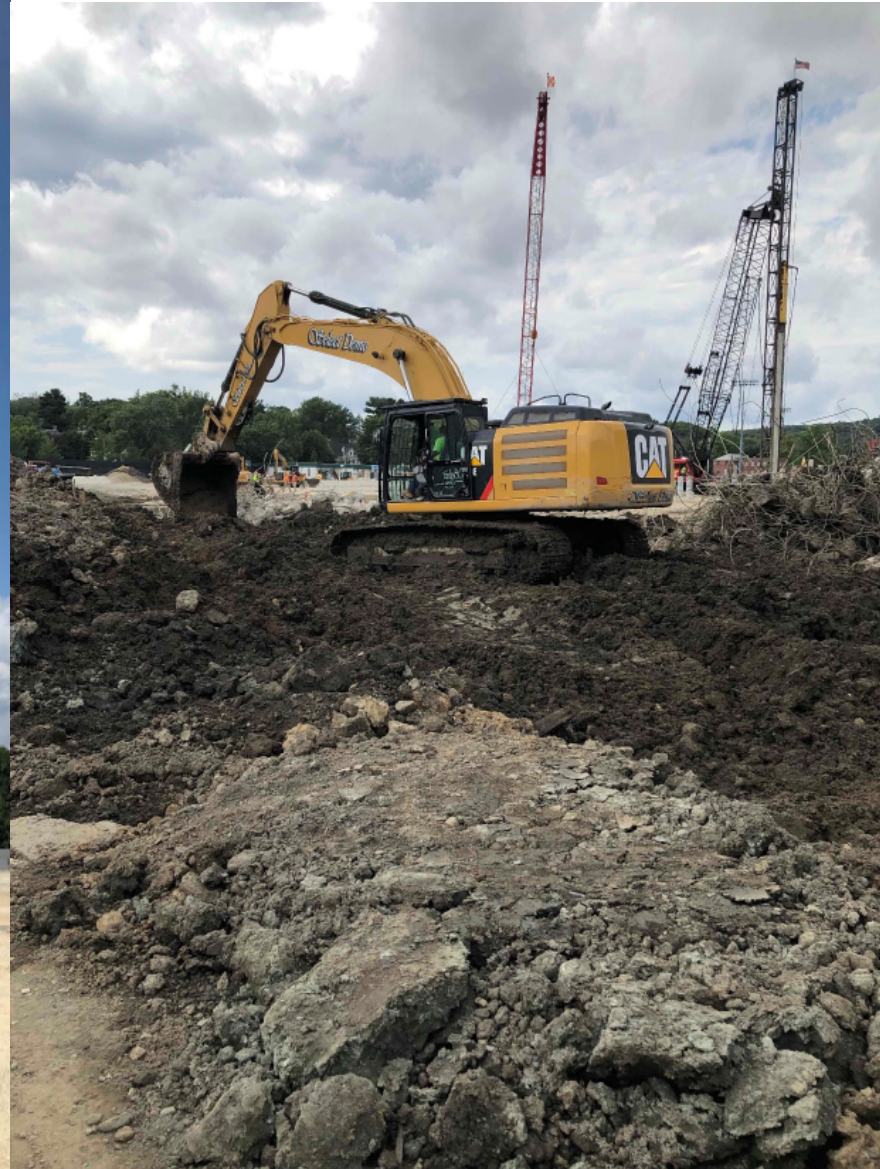
Photo 5 - Completion of Foundation Removal.
