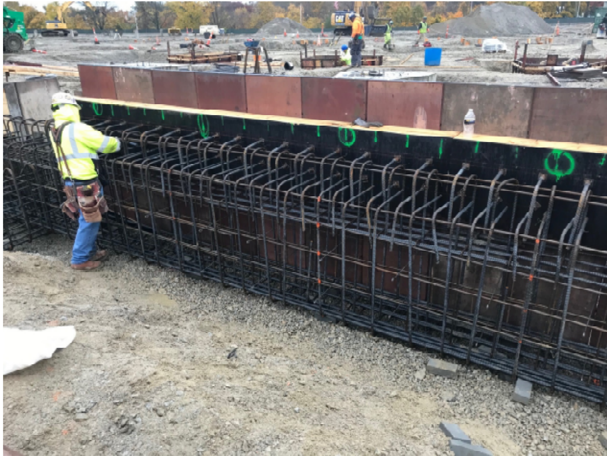
Photo 2 – Installation of Grade-Beam Rebar and Brick Shelf Rebar.
