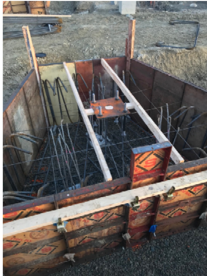
Photo 3 – Formed and Reinforced Pile Cap with Anchor Bolts.
