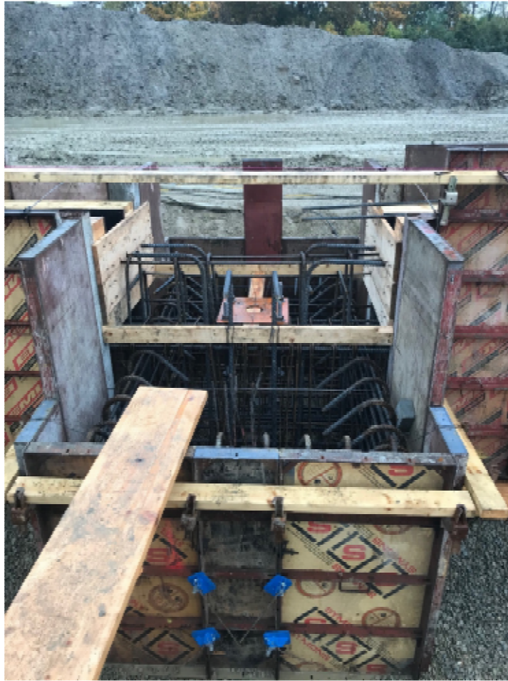
Photo 4 – Exterior Pile Cap at Grade Beam with Anchor Bolts.
