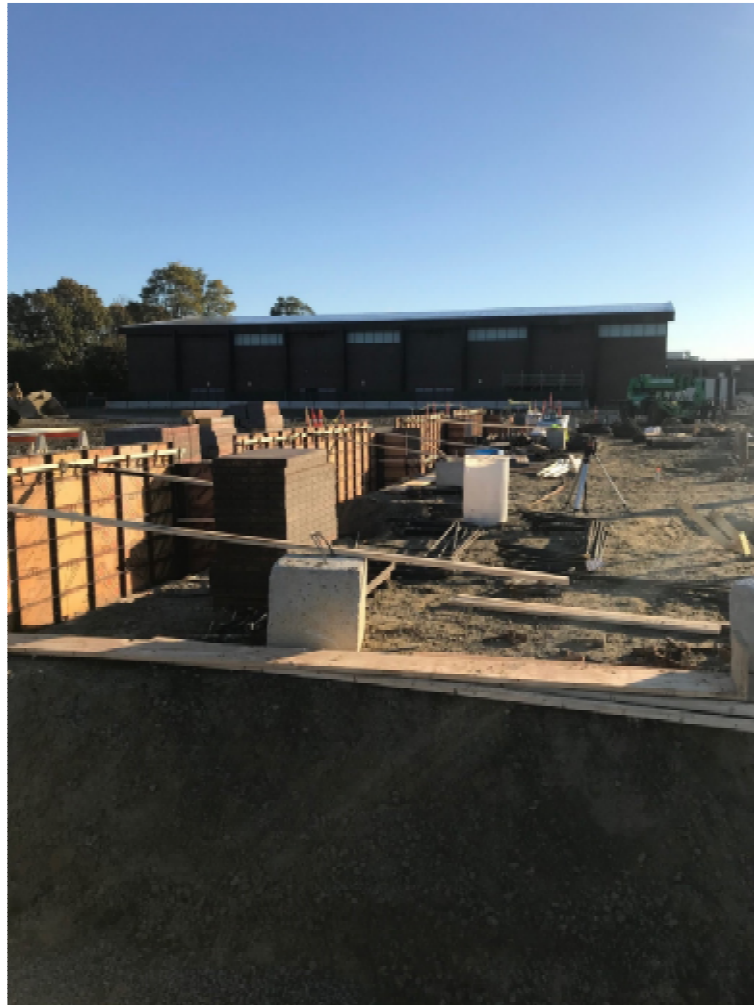
Photo 1 – Installation of Concrete Formwork.
