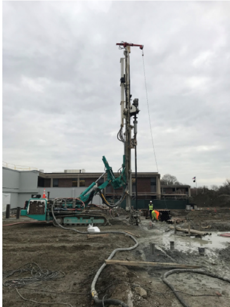
Photo 1 – Installation of Drilled Mini-Piles.
