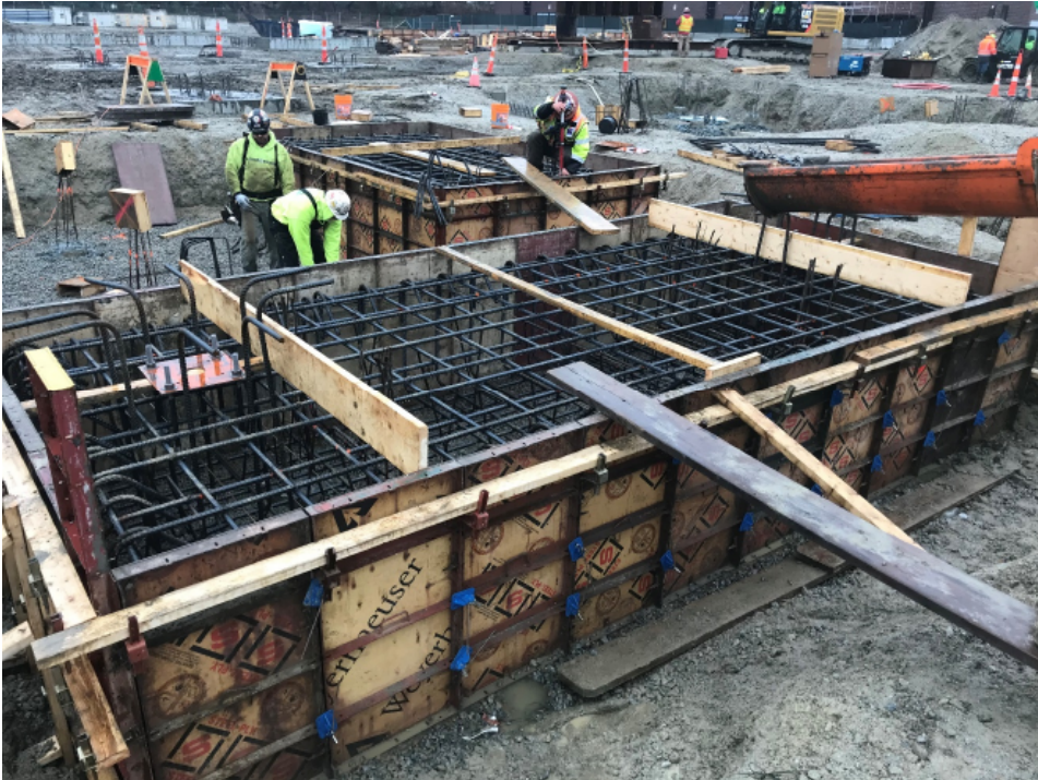
Photo 4 – Interior Pile Cap at Grade Beam with Anchor Bolts.
