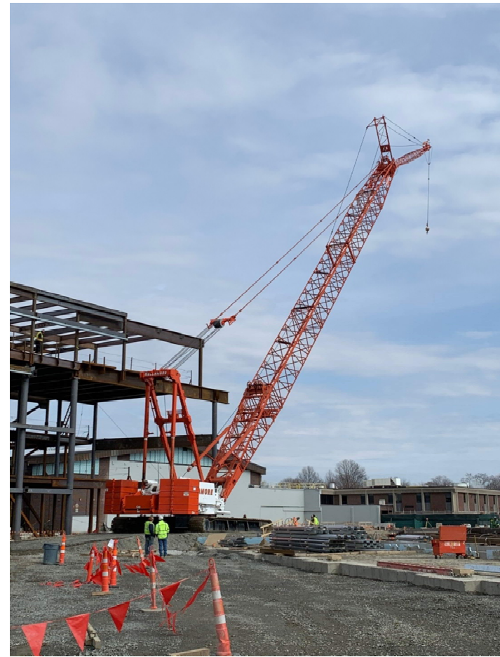
Photo 6 – Moving 2250 Crane into Area C/D to Start Steel Erection.
