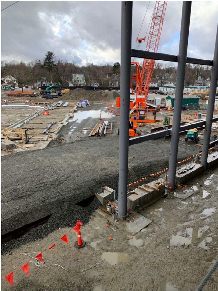
Photo 5 – Temporary Ramp to Drive 2250 Crane Over Area A Foundation Wall.
