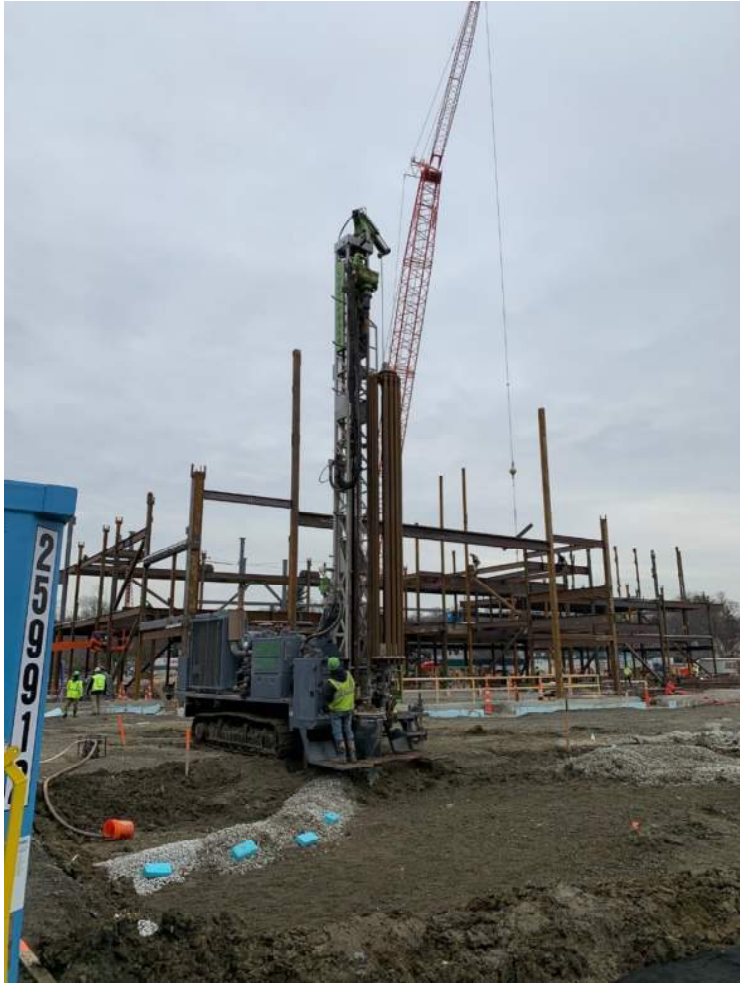
Photo 1 – Start of Geothermal Well Drilling
