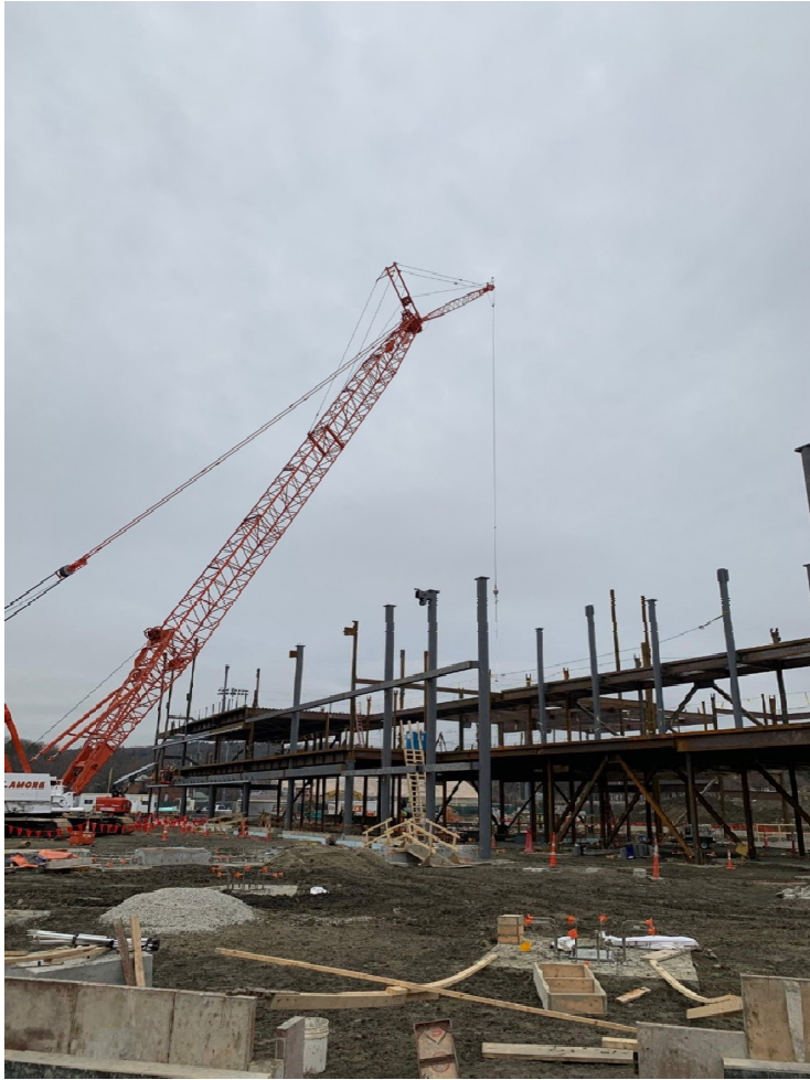
Photo 3 – Steel Erection of Area B Showing Level 2 through Level 3 Framing.
