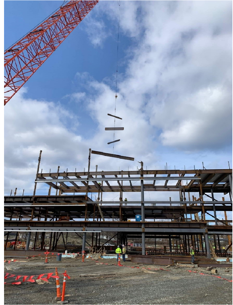
Photo 4 – Erection of Area B Framing From Level 2 through Level 4.
