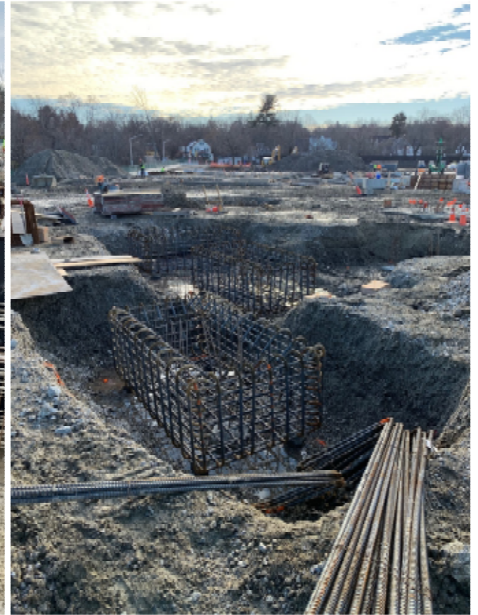
Photo 6 – Rebar Installation in Area C.
