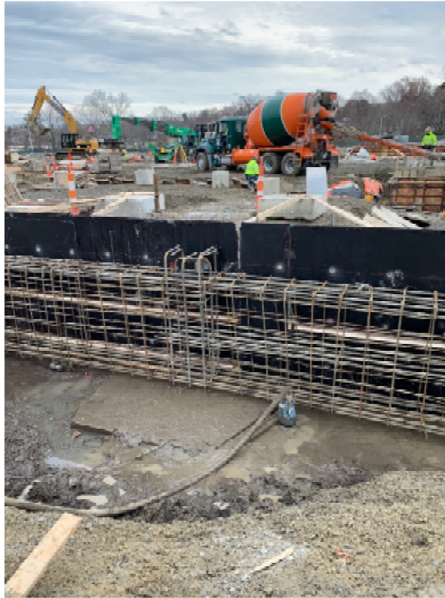
Photo 5 – Auditorium Stage Grade Beam with Water Stop.
