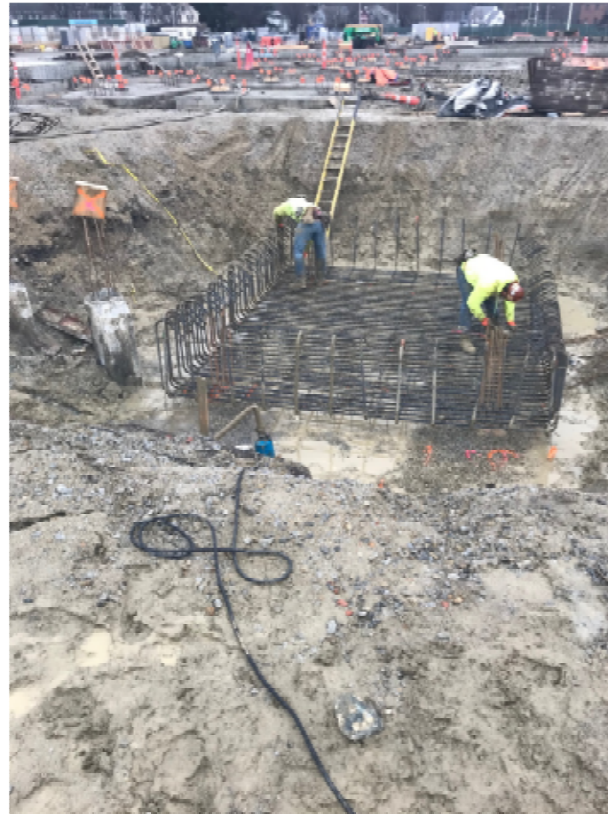
Photo 3 – Progress of Rebar Installation for Area B Elevator Pit Pile Cap.
