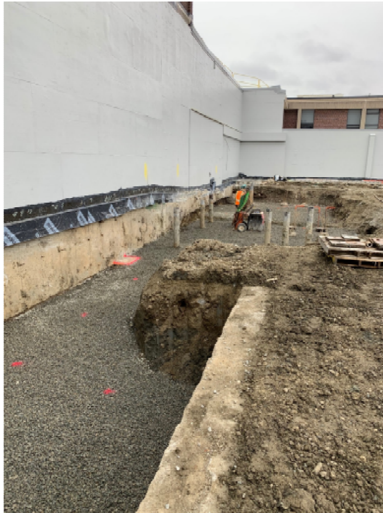
Photo 1 – Cutting and Detailing of Drilled Mini-Piles.
