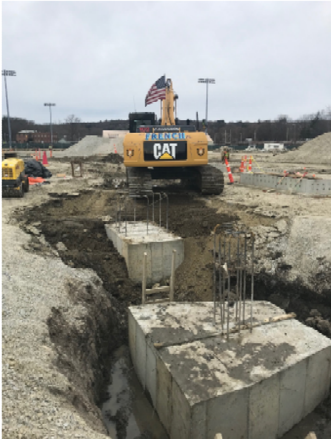
Photo 4 – Auditorium Stage Pile Cap Installation with Pier Rebar.
