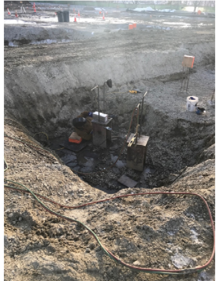
Photo 2 – Cutting and Detailing of Steel H-Piles.
