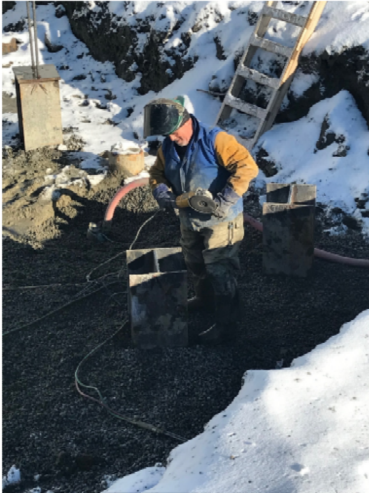
Photo 2 – Cutting and Detailing of Steel H-Piles.
