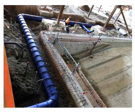
Photo 2: Installation of vapor barrier and rebar in preparation of pouring slab on grade in area C
