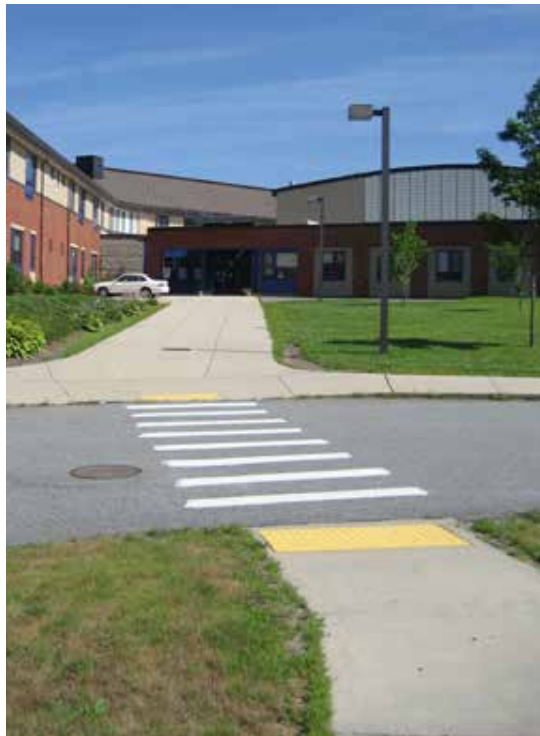
Marked crosswalk (continental design) across a campus driveway
