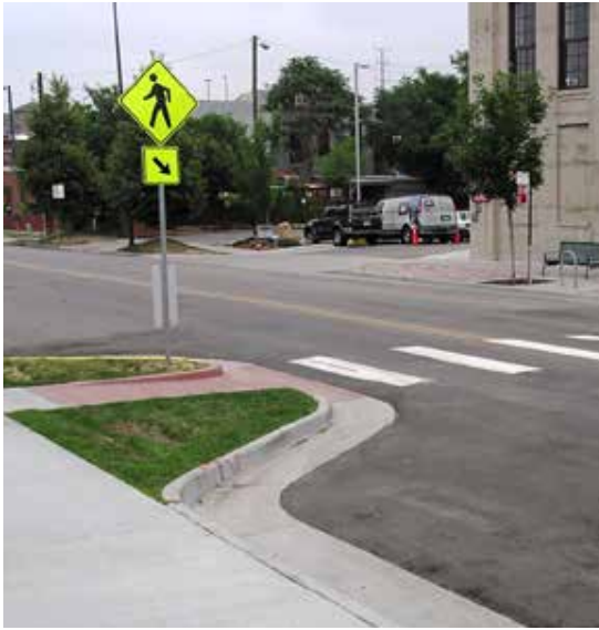
Curb extension at a mid-block crossing
