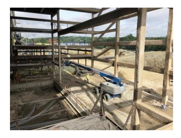
Photo 5 – Building A Corridor with MEP components, wall framing, and some sheathing installed.
