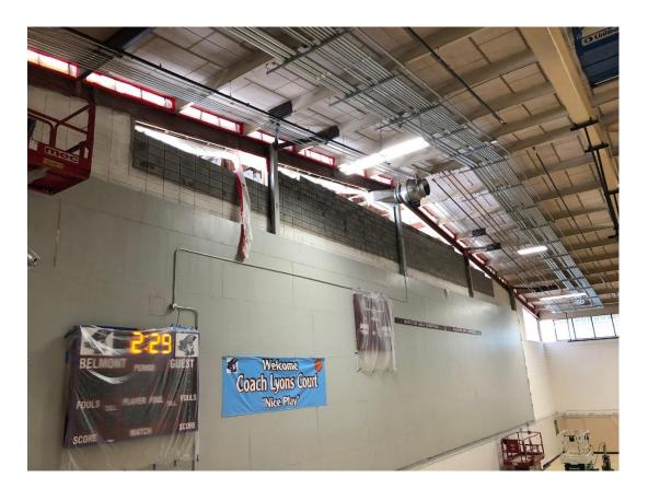
Photo 9 – Plumbers Install Roof Drains; Pipe-Fitters Install Fire Protection Piping.
