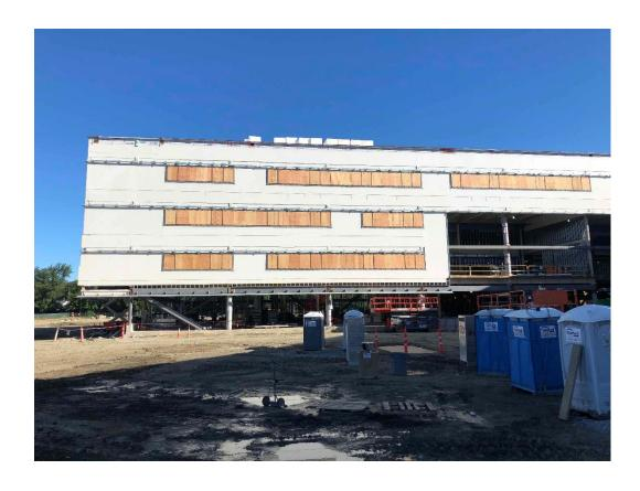
Photo 7 – Brick Installation at Building A East and Sheathing Installation at Building C South.
