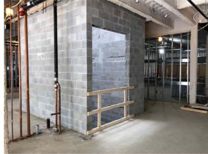
Photo 6 – Elevator Shaft in Area B
