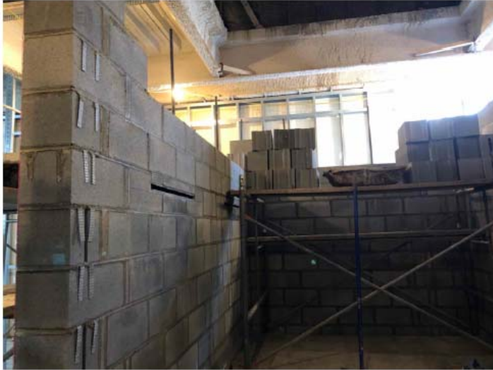
Photo 5 – Installation of Elevator Shaft Area B
