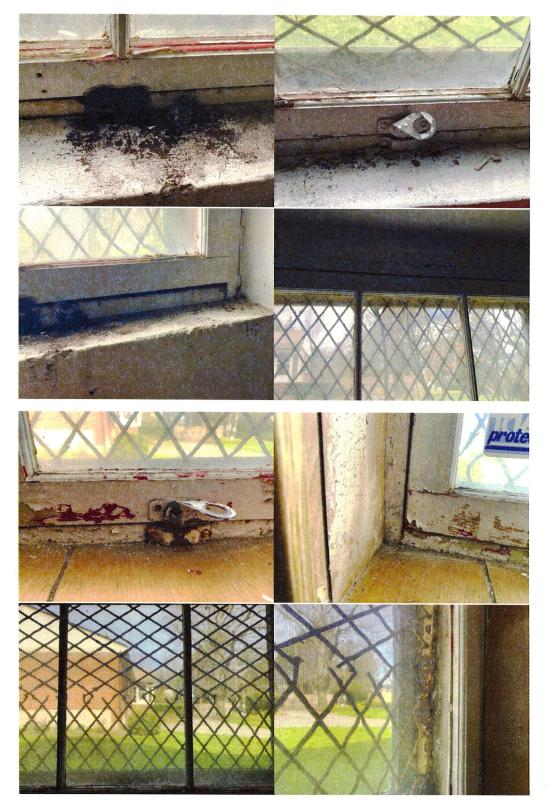
Black mold, metal decayed, wood rotten, frame at joints swollen due to water damage. Window, not fitting frames. Latches are not functioning for security.
