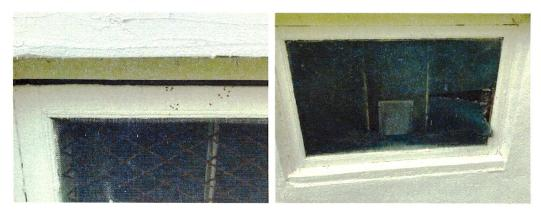
The outside view shows **windows separating from the frame and letting in outdoor elements**, screening torn and not closing correctly, leading to energy loss and a security risk. Windows are currently not openable.
