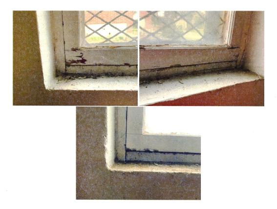
Framework separating at joints, window wood expansion/rot, ill-fitting and not closing correctly or opening at all, hinge broken, grill rusted.
