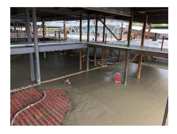
Photo 3 – Area C Radiant Piping Prior to Slab on Deck Placement.
