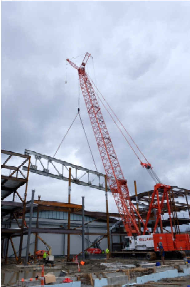
Photo 4 – Erecting 32 Ton Truss in the C/D Wing.
