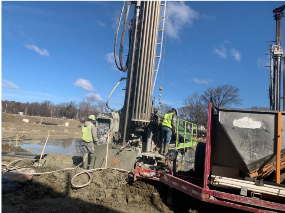
Photo 6 – Continuing Geothermal Drilling in Field #1.
