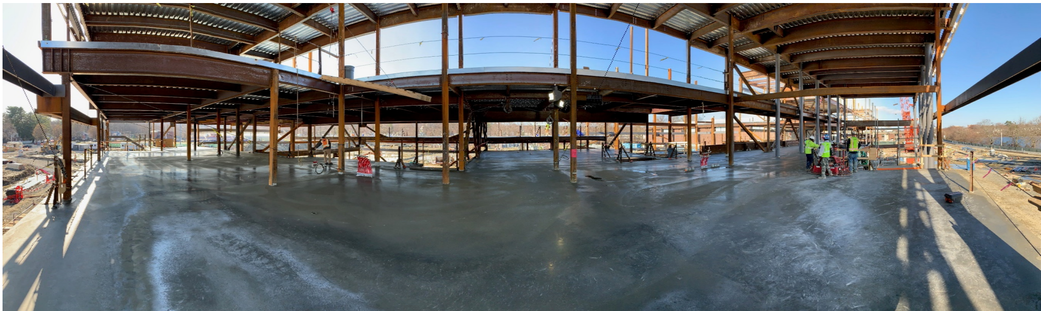
Photo 3 – Level 2 Area B Concrete Placement
