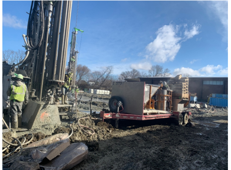
Photo 7 – Grouting Geothermal Well.
