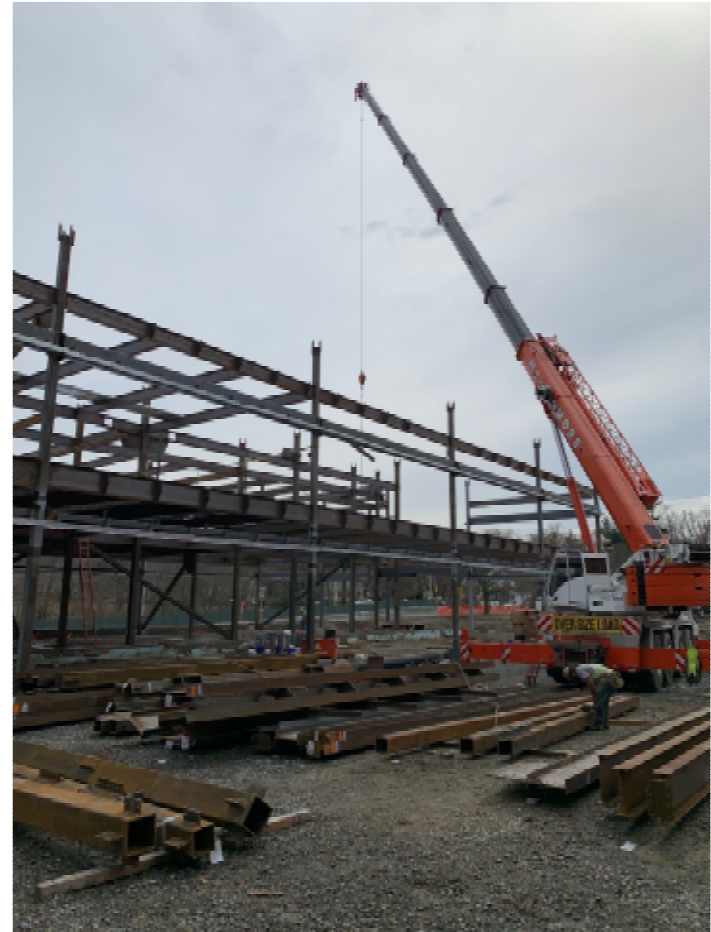
Photo 5 – Erecting Steel in Area A Wing.
