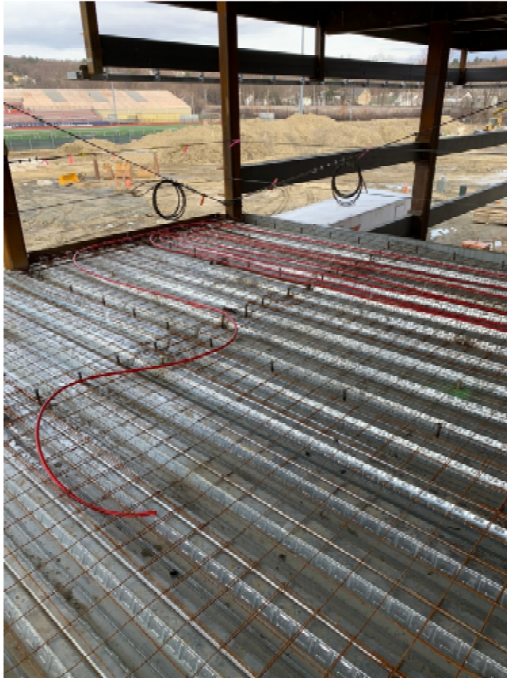
Photo 1 – Start of Radiant Tubing Installation.
