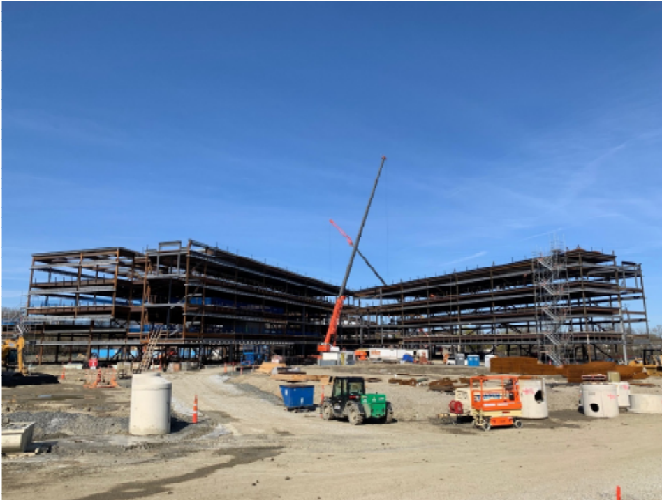
Photo 7 – Building A and B Erection Completed.
