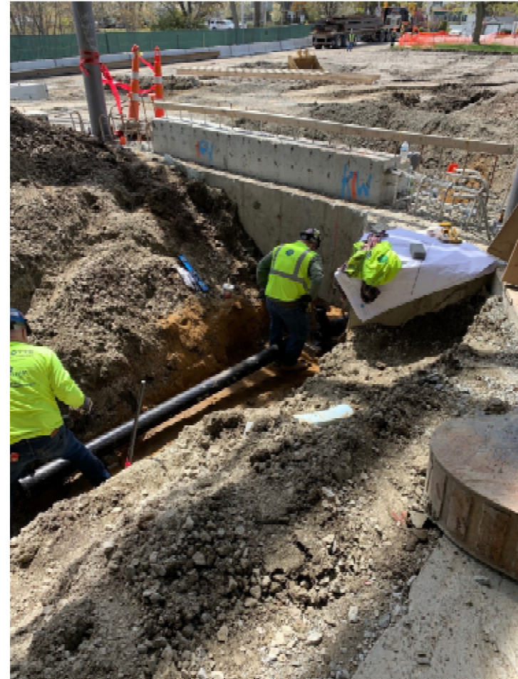
Photo 8 – Under-slab Utility Work in Building A.
