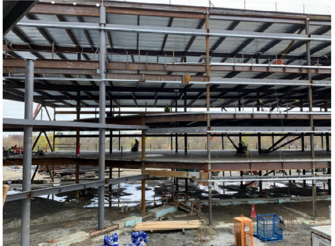
Photo 4 – Finishing Level 2 Building A Slab.
