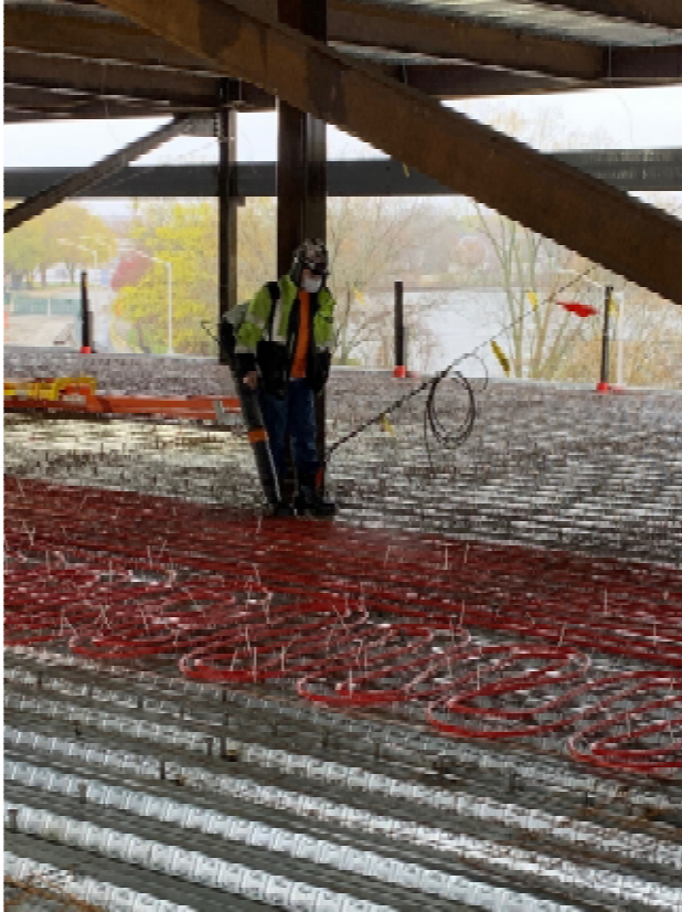
Photo 5 – Radiant Tubing Installed Within Slab on Metal Deck.
