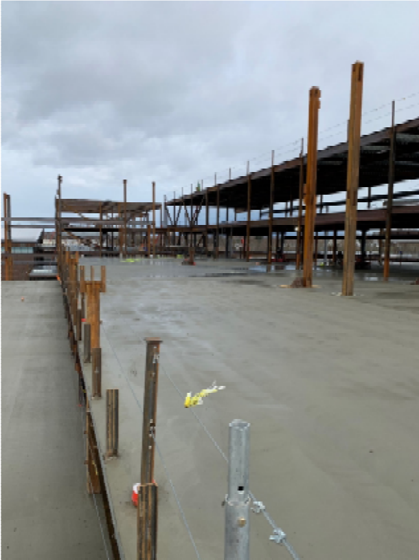
Photo 3 – Finishing Level 3 Building B Slab.
