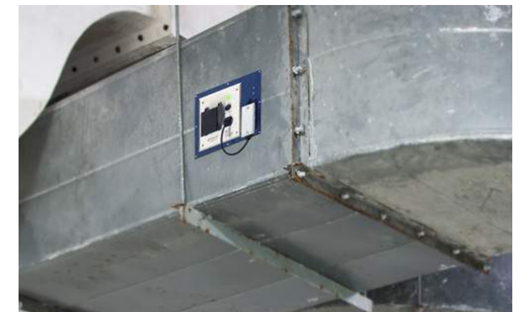
Bipolar Ionization Applied to Duct
