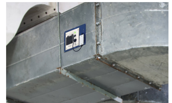
Bipolar Ionization Applied to Duct
