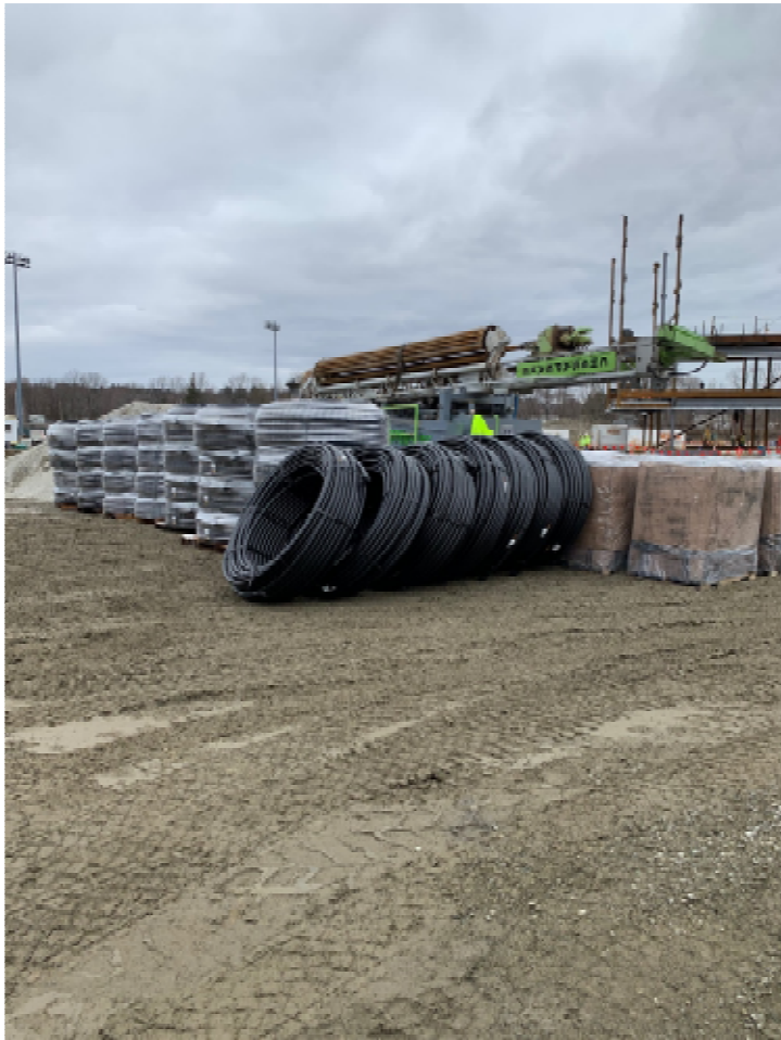
Photo 9 – Geothermal Piping Coils, Grout and Drill Rig.
