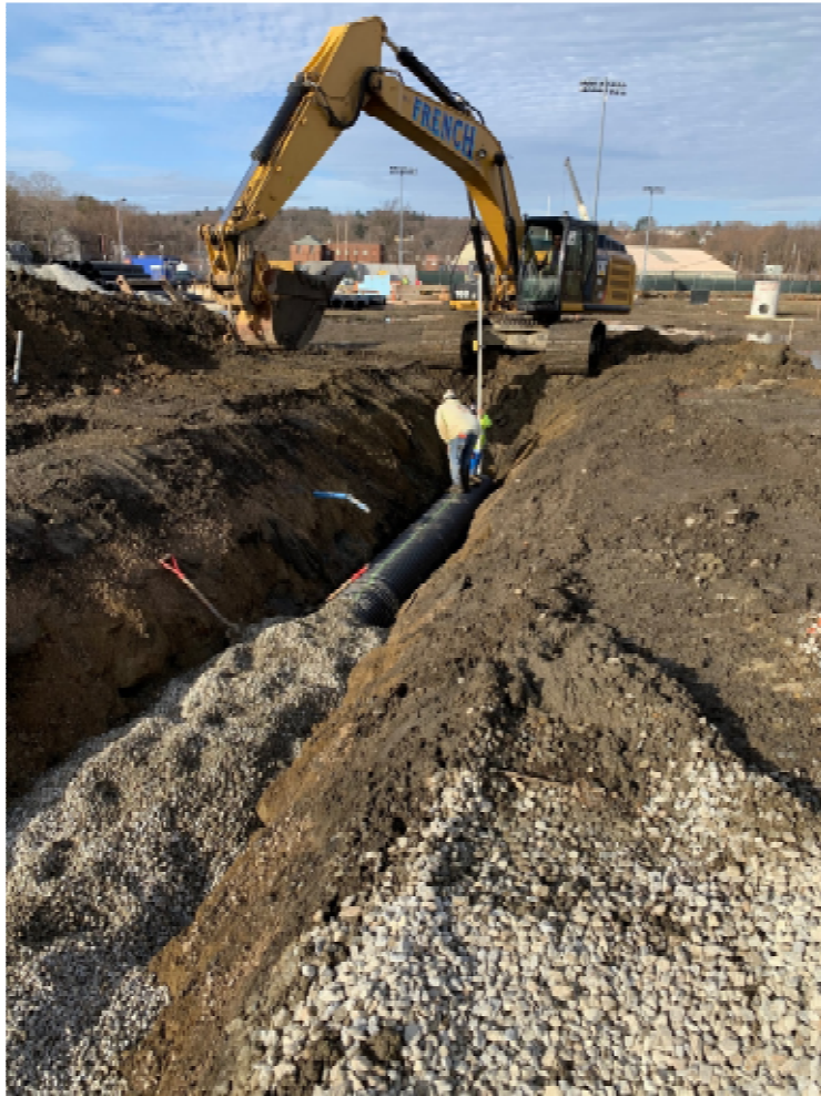
Photo 5 – Progress of Drainage Piping Installation.
