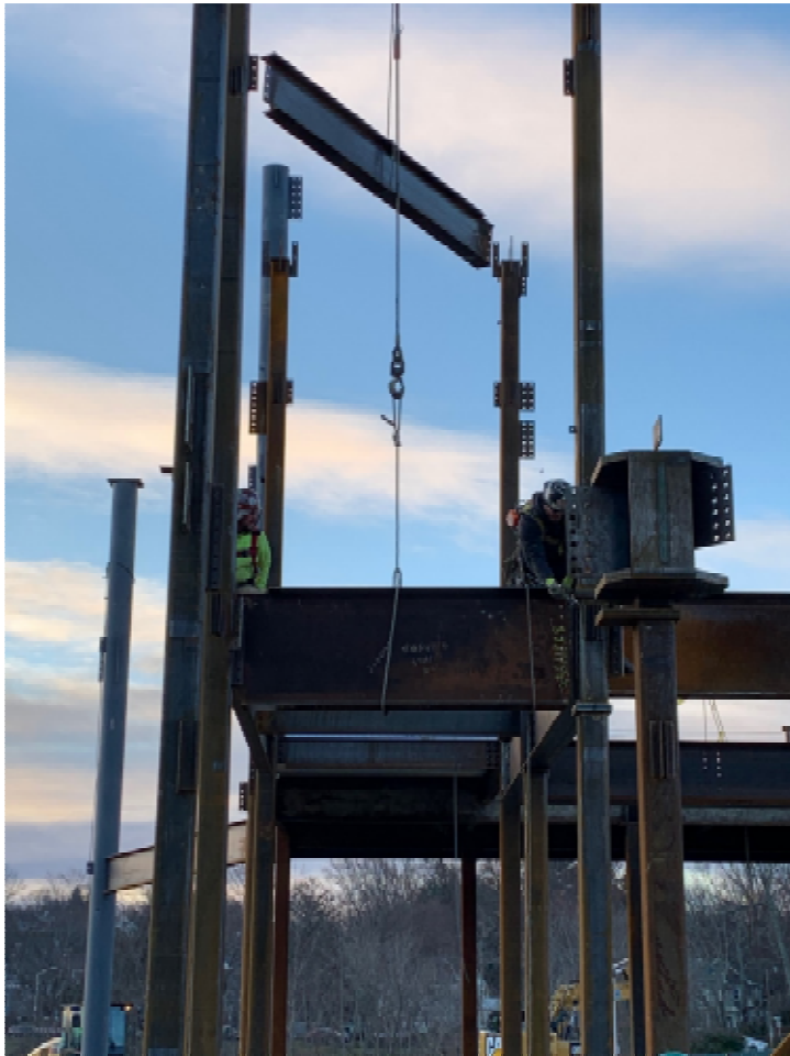
Photo 7 – Structural Steel Install in Auditorium.
