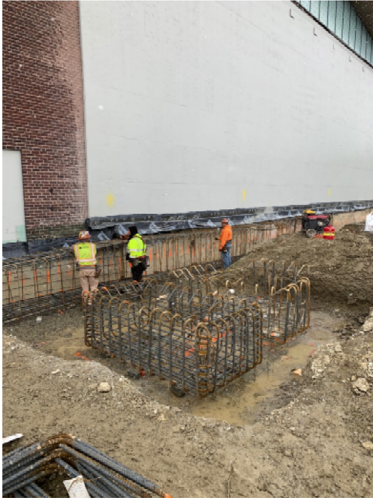
Photo 1 – Reinforcing Pile Caps and Grade Beams in Area C.
