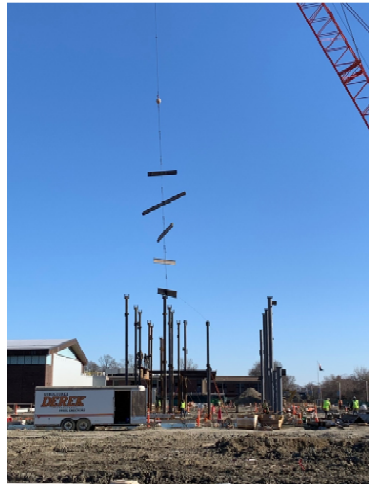
Photo 8 – Structural Steel Installation.
