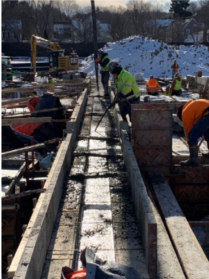
Photo 3 – Concrete Placement in Area A.
