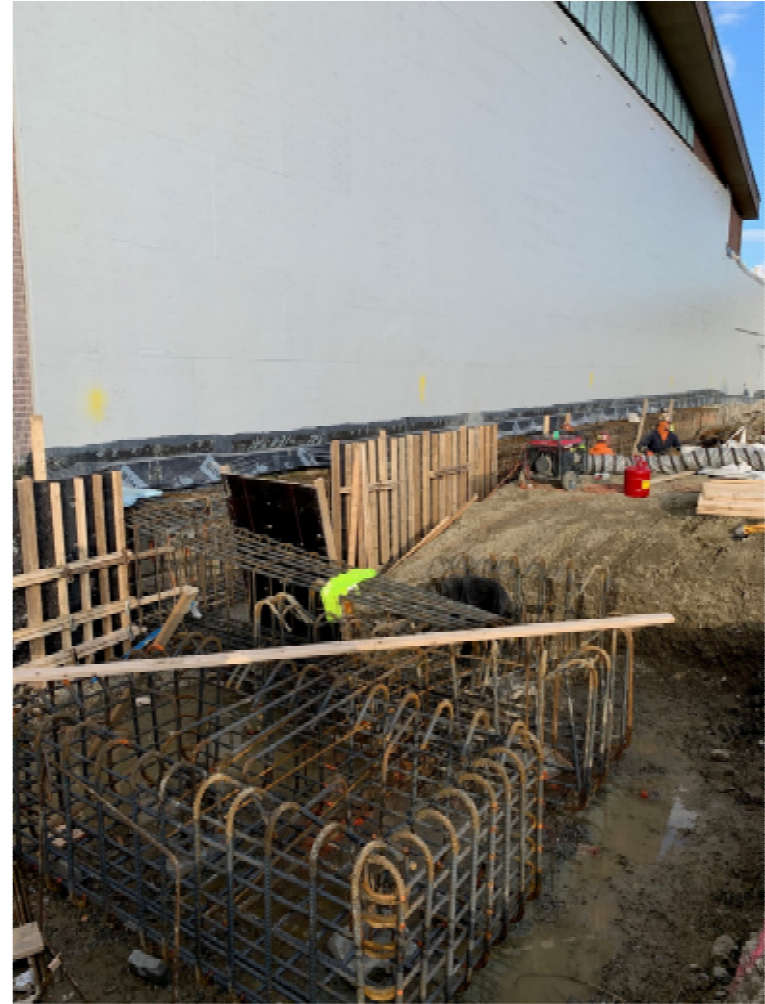
Photo 2 – Forming Pile Caps and Grade Beams in Area C.
