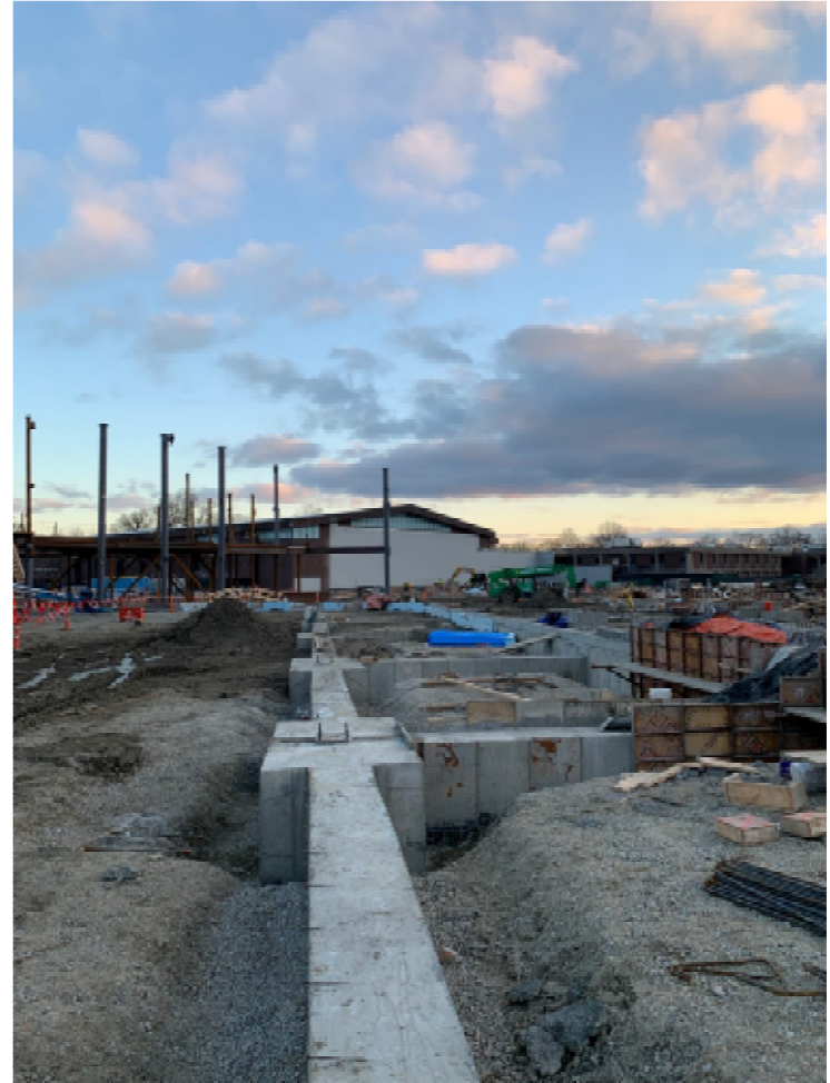
Photo 4 – Concrete Progress in Area A.
