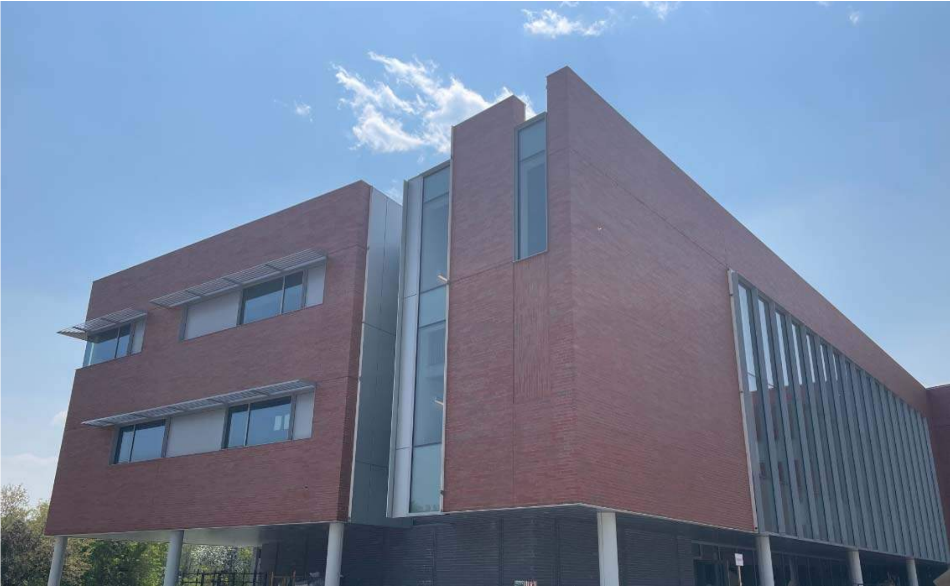
Area D Façade
