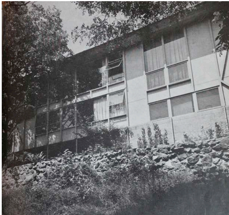
View of original fenestration
