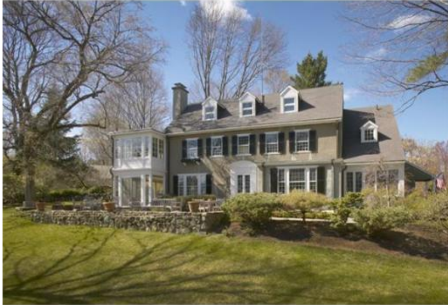
Web Photo of Rear elevation
