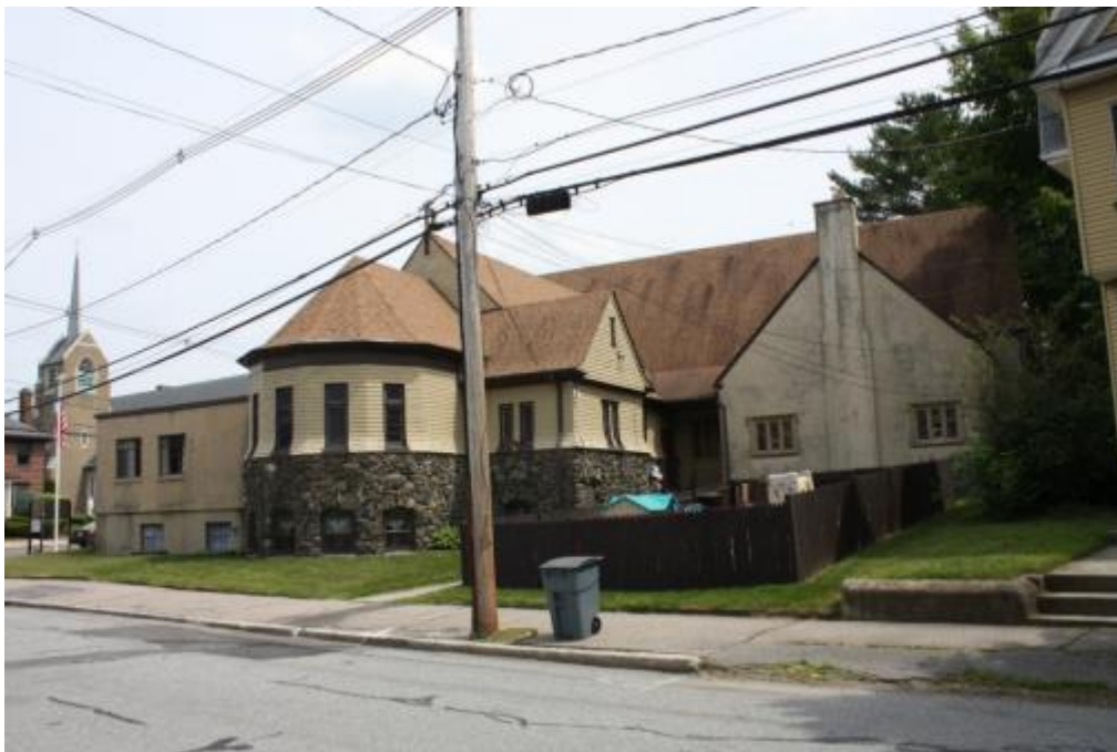
View from Burnham Street showing original Shingle Style chapel at center, 1955 to left and 1935 at right.
