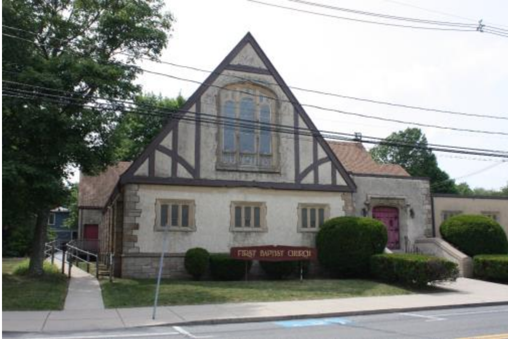
1935 Addition, Lexington Street façade
