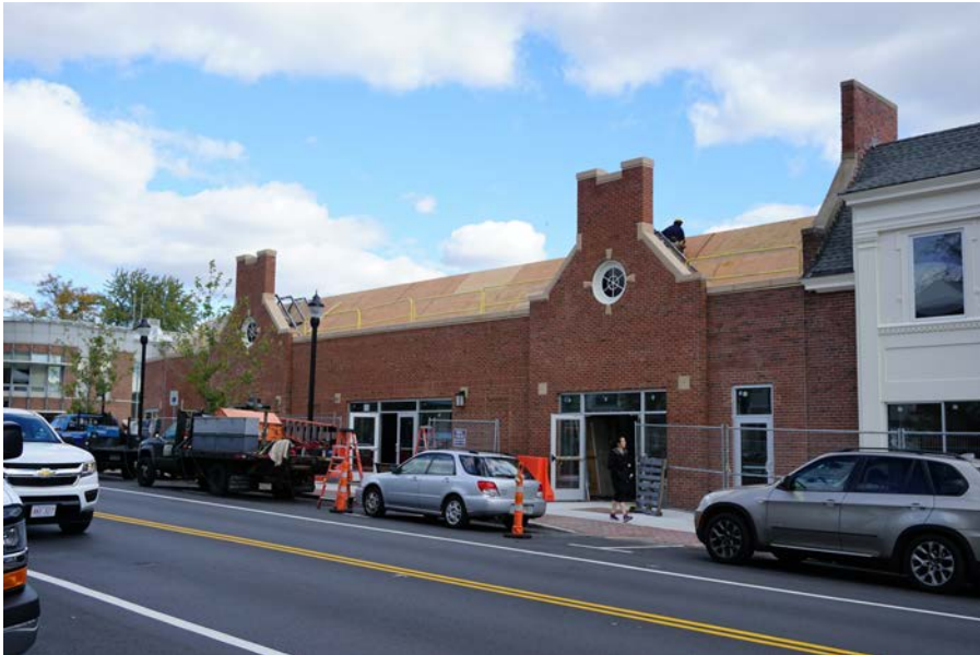
Work in progress (Oct. 2016)
