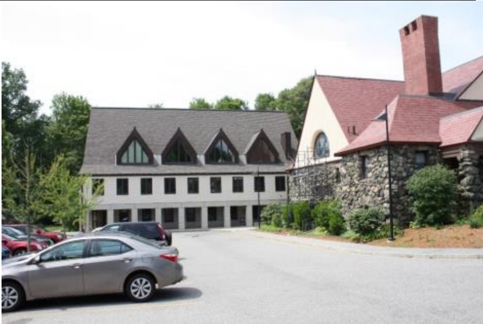
North façade of 2004 Parish Hall and Classroom addition
