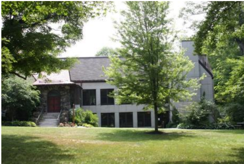
West elevation of 2004 Parish Hall and Classroom addition
