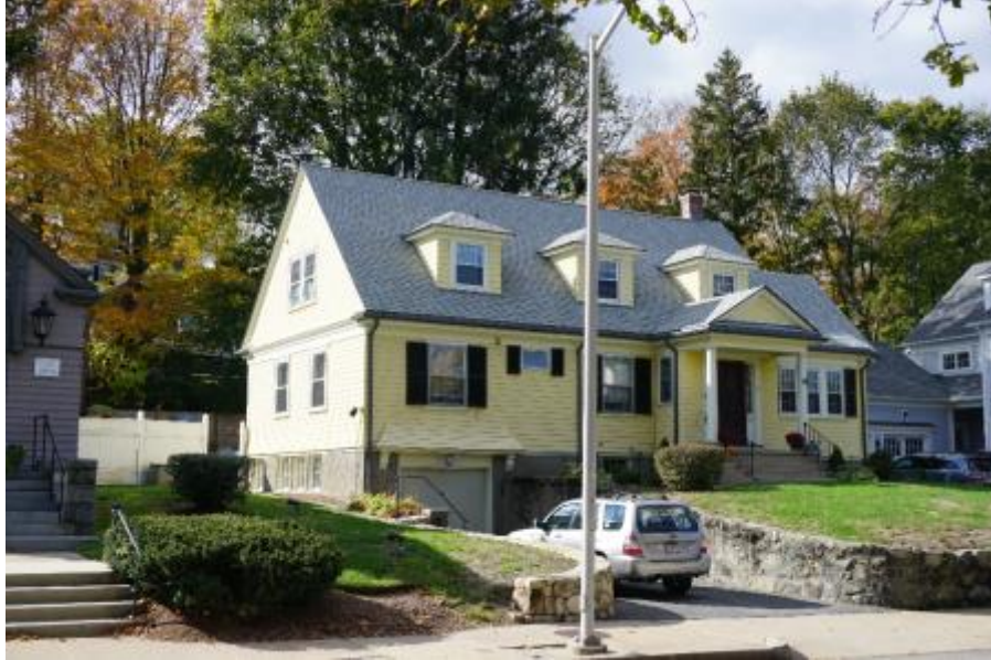
Rectory at 65 Common Street (BLM.313)
