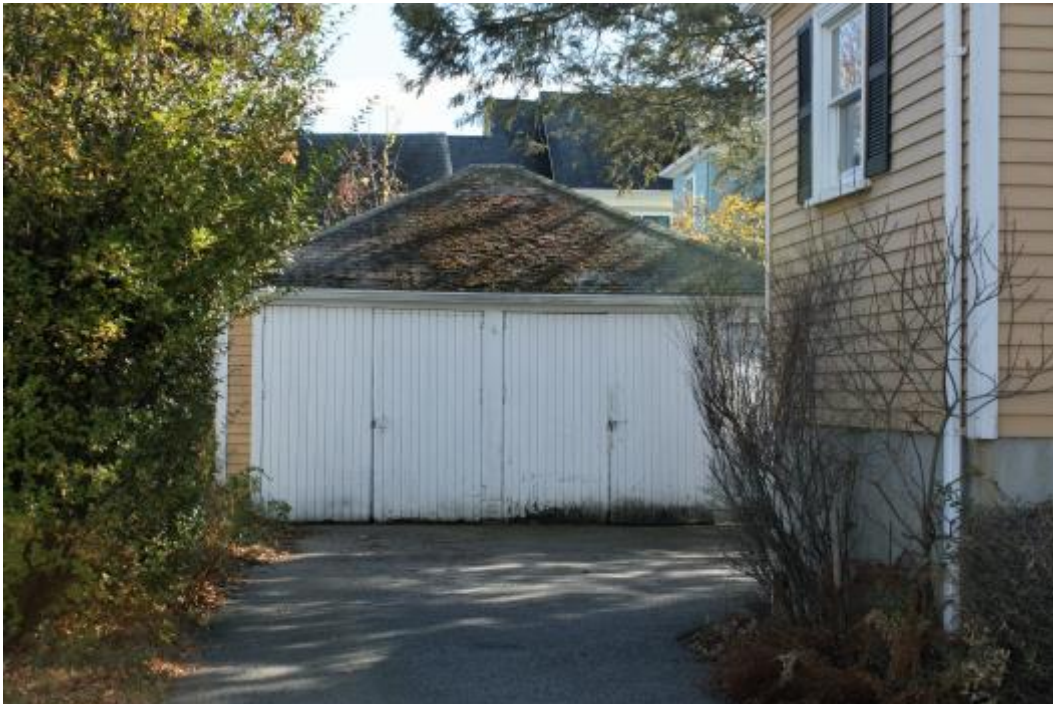
Garage (1922) facing Waverley Street
