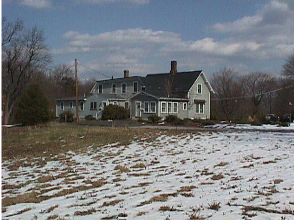
View of Rear elevation
