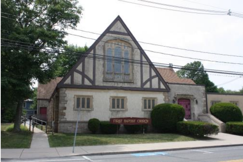
1935 Addition, Lexington Street façade
