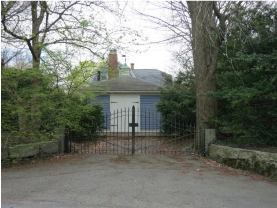
Shed, view from Clark Street
