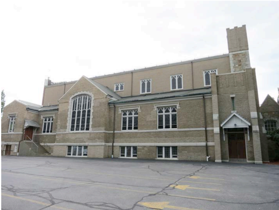
North elevation of Church
