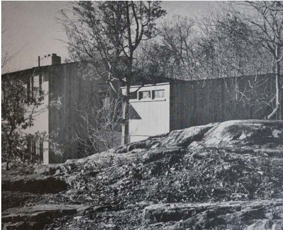
Northeast corner of house
