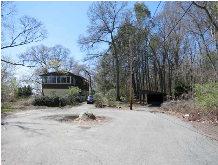
View looking SW at house (left) and carport (right)
