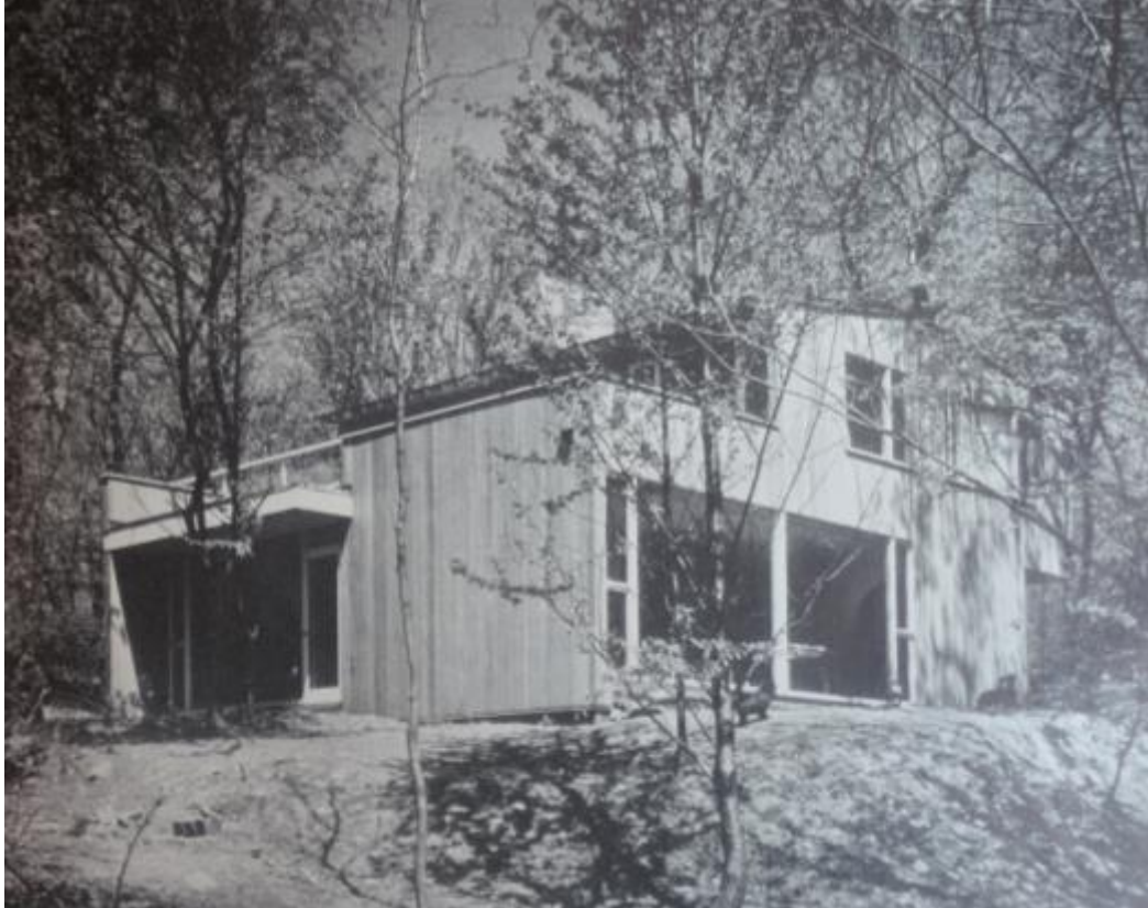
Gordon House, 1941 (looking north)
