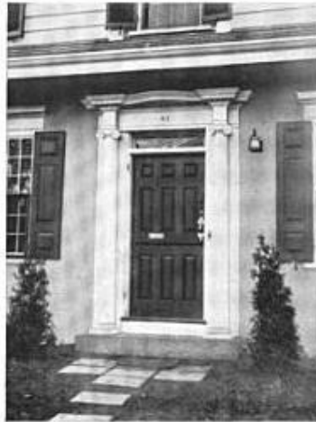
Showing the front door and wooden shutters.
