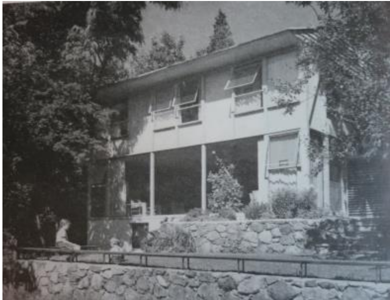
Original southeast elevation
