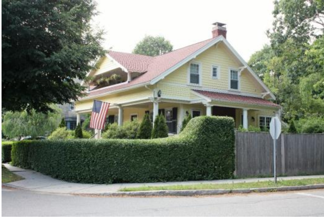
Current view of south façade and east elevation.
