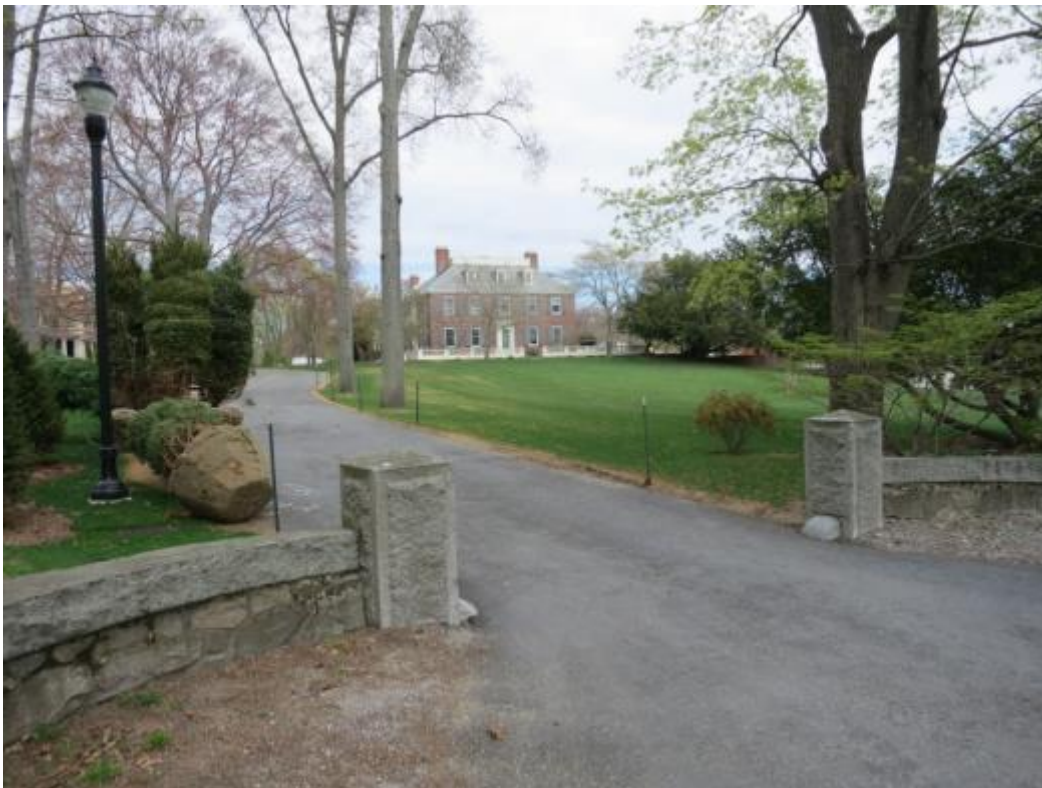
Driveway Entrance on Concord Avenue
