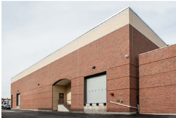
Front side of the completed Blair Pond Substation in late 2016.
