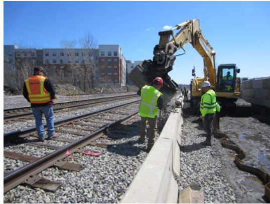
Sheeting installation as part of the Transmission line project in April 2016.
