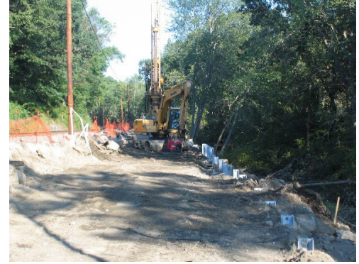
Rail-with-trail Retaining Wall Construction in Lincoln, RI
