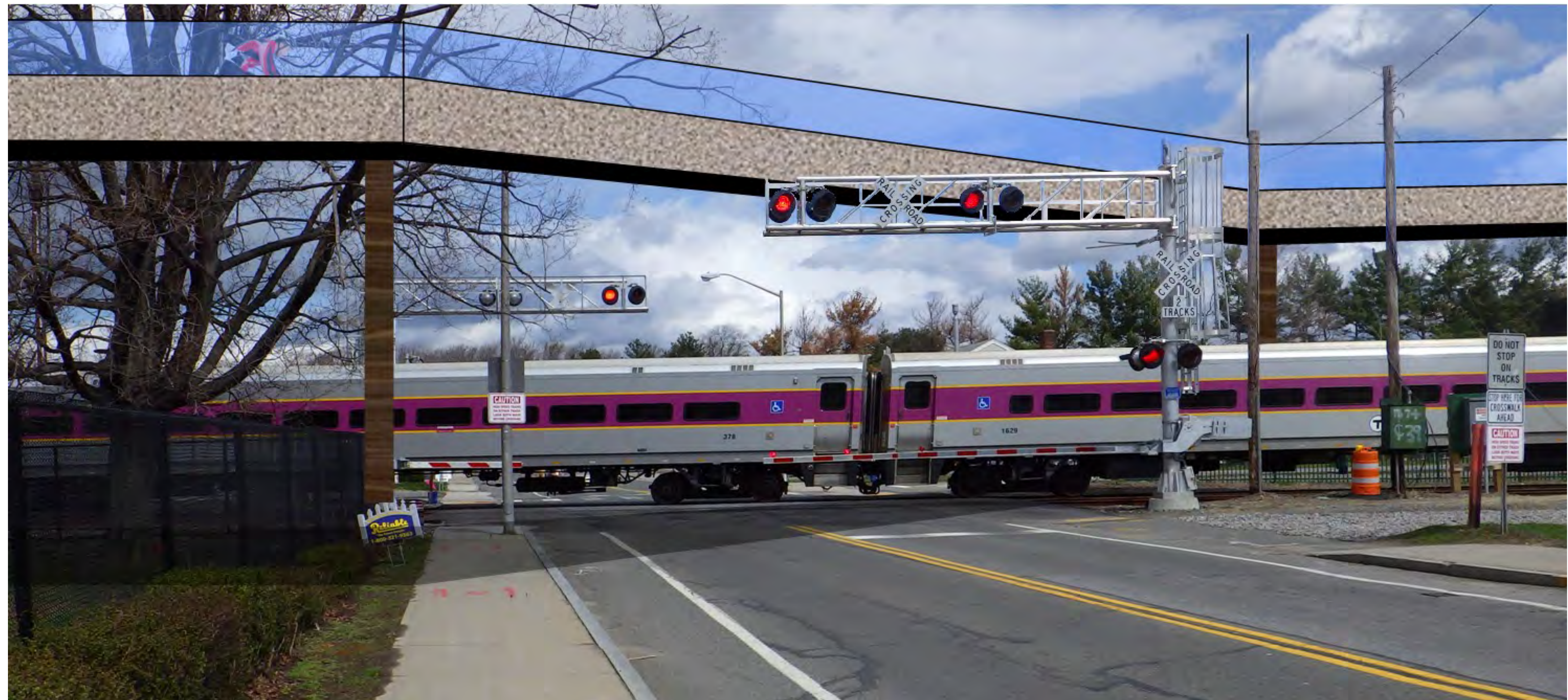
Cross Brighton Street and Rail (E4c): Elevate to 24' west of Brighton Street and cross road/rail diagonally. Impacts building southwest of road/rail intersection.
