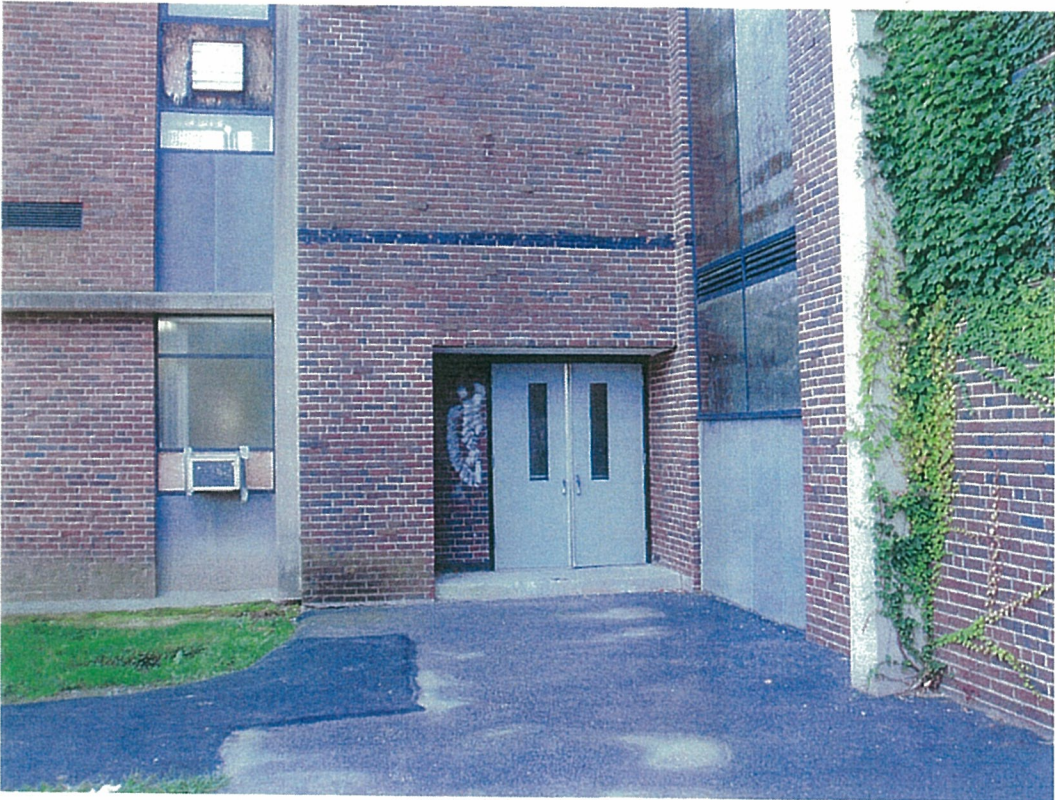
REAR ENTRANCE TO FIELD HOUSE LOBBY
