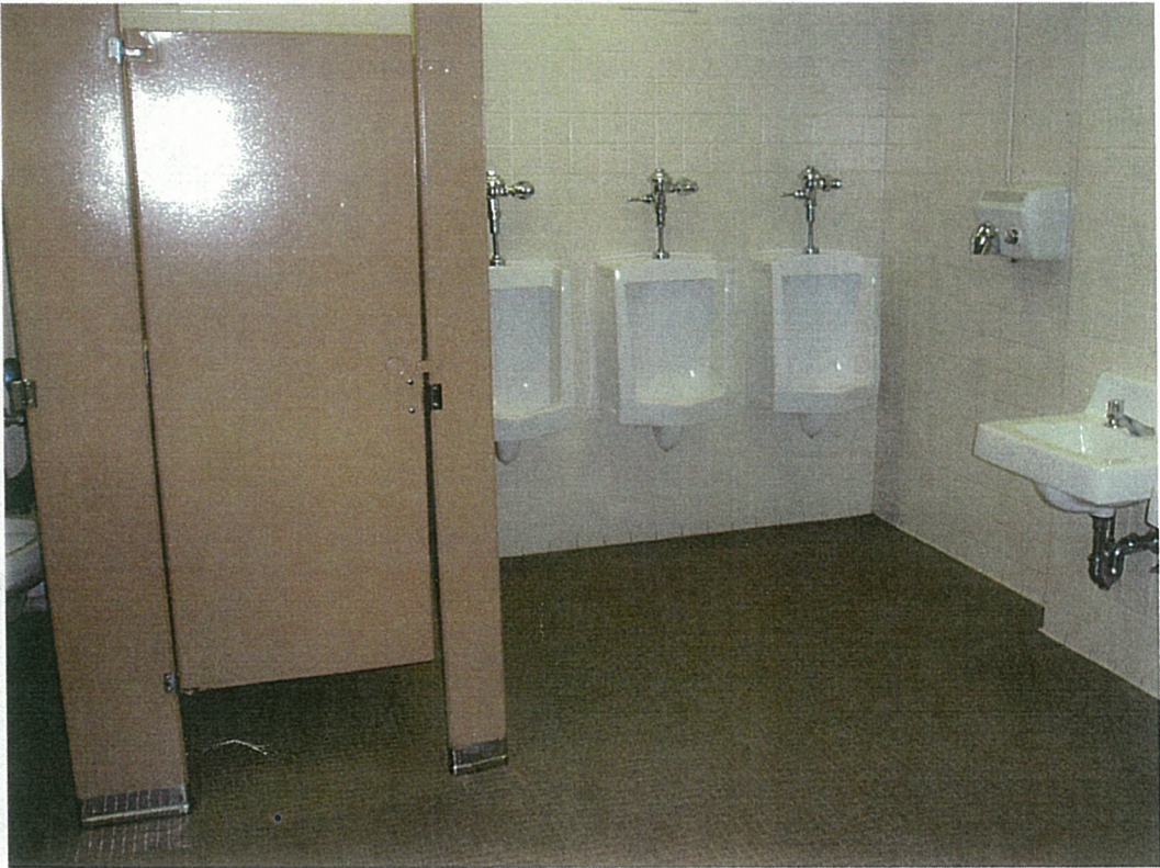
LOCKER ROOM TOILETS
