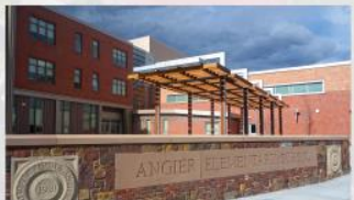
Newton School Building Program Projected Completion Winter 2019 Architect: DiNisco Design Partnership & Perkins Eastman CM: WT Rich Grades: K-5 Cost: $122.5M
