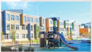
Milford Woodland Elementary School Projected Completion Fall 2016 Architect: HMFH Architects CM: Shawmut Design & Construction Grades: 3-5 Cost: $60.9M
