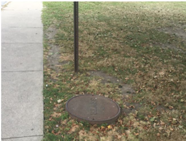
Figure 2: Sewer Manhole along the south of the School
