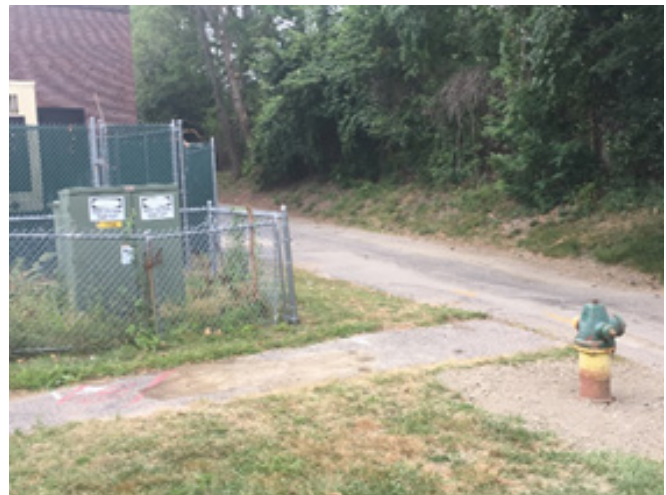
Figure 5: Fire Hydrant along the north of the School
