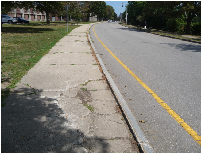
Sidewalk in poor condition looking east up drop-off loop (left and right); Informal footpath around Claypit Pond (right)
