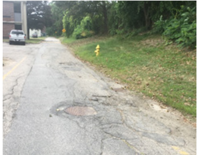
Figure 4: Fire Hydrant along the west of the School
