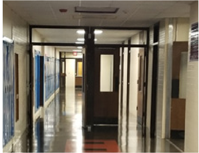
Figure 5: 29.5" Wide Cross Corridor Doors
