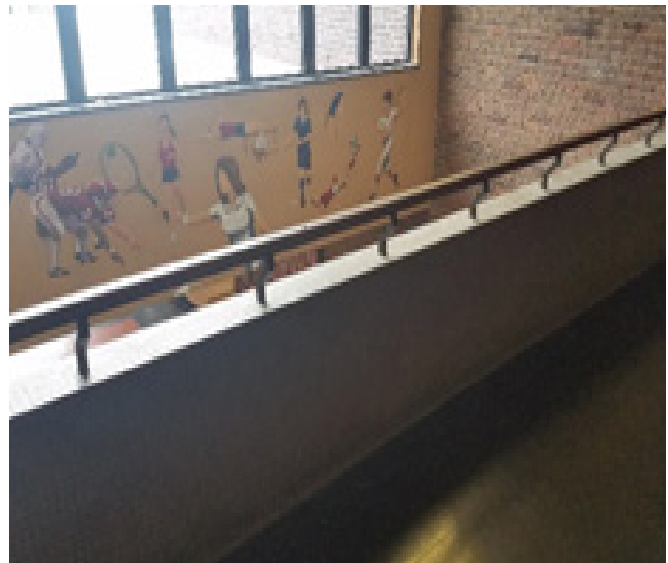
Figure 6: 2-Story Opening with 35.5" Guard
