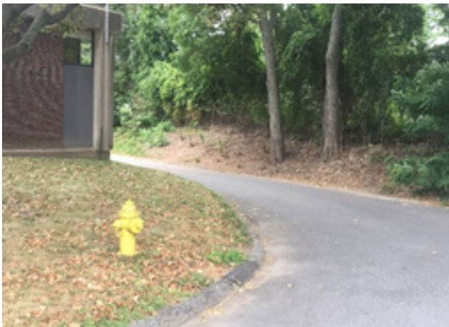
Figure 3: Fire Hydrant along the north of the School
