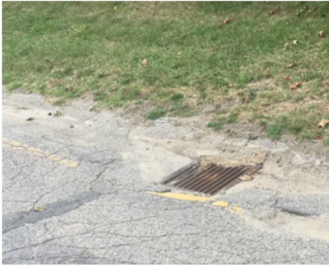
Figure 1: Catch Basin along the north of the School
