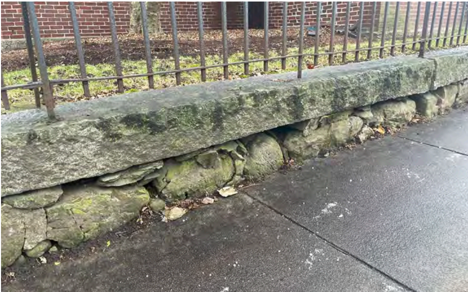
Images of the granite block retaining wall and iron picket fence along Huron Avenue and Grove Street
