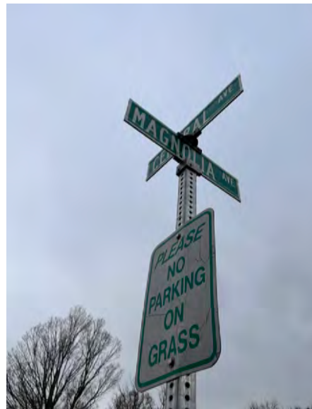
Signs with more modern aesthetics in the Cemetery, (left) drive naming sign: aluminum sign on square galvanized steel posts, and (center): street and rules signs
