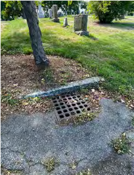
(top) Condition of drives and (bottom) curbing in the Cemetery (left to right) granite curb at catch basin, recycled concrete curb painted white, and bituminous concrete curb
