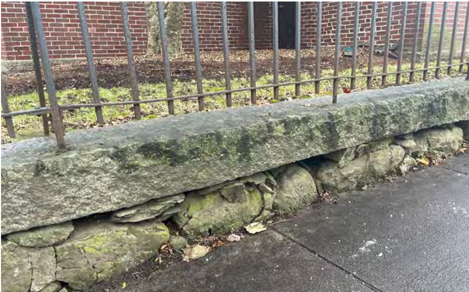
Boundary wall along Huron Avenue
