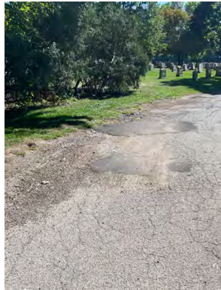
Depressions and filled pot holes on Goldenrod Path
