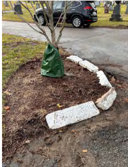
(top) Condition of drives and (bottom) curbing in the Cemetery (left to right) granite curb at catch basin, recycled concrete curb painted white, and bituminous concrete curb
