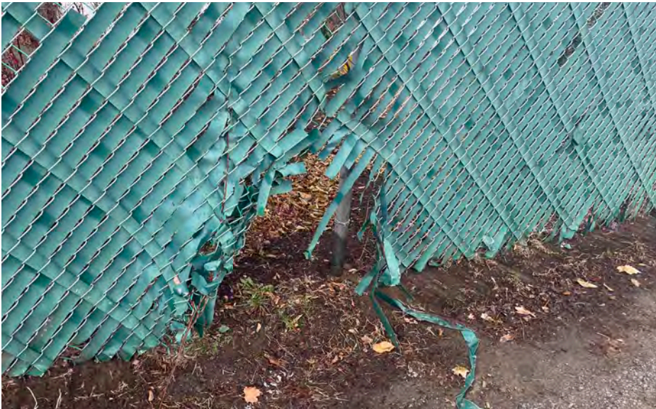
Chain link fence fabric and privacy slats have been cut, presumably to allow dogs into the Cemetery.
