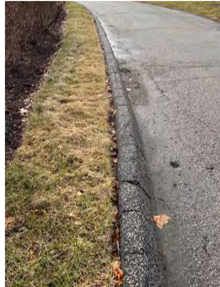
(top) Condition of drives and (bottom) curbing in the Cemetery (left to right) granite curb at catch basin, recycled concrete curb painted white, and bituminous concrete curb
