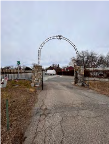
Block cracking at entry and on Central Avenue (as well as edge cracking)
