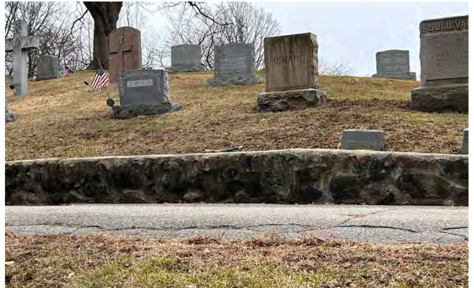
Retaining wall above Huron Avenue
