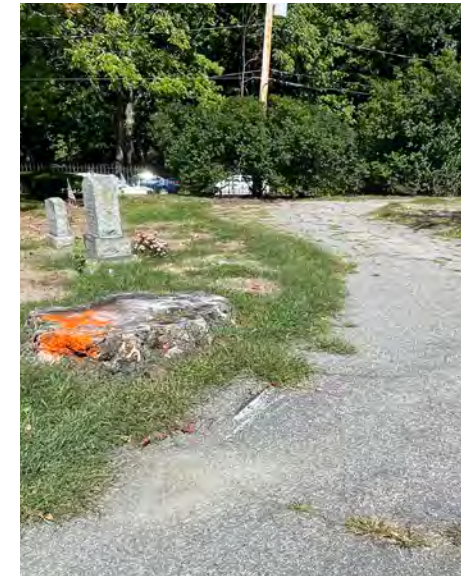
Plow scars and root upheaval on Iris Avenue
