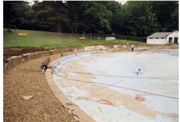
Deck Replacement and tank repairs 1995
