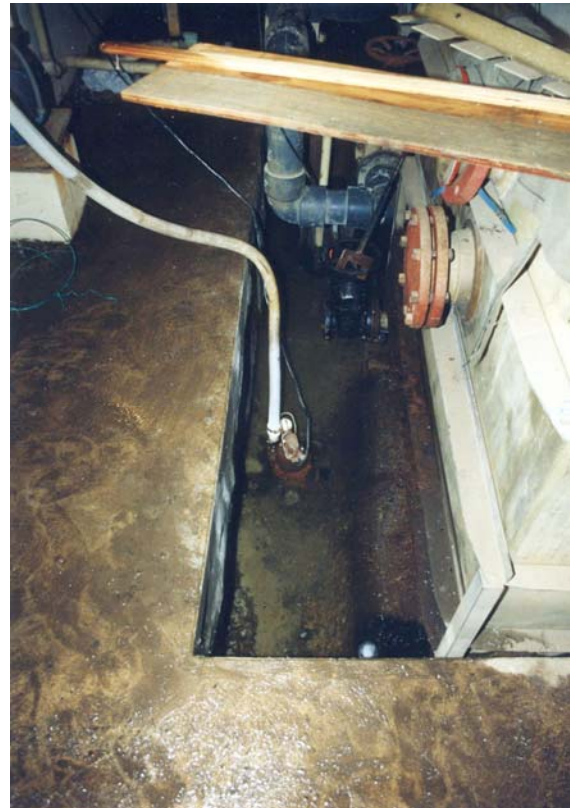
Submersible Pump in Operation to remove ground water
