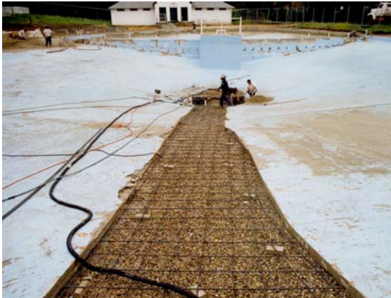
Installation of Main Drain Lines in 1995
