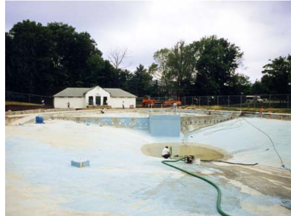
Pool Repairs in 1995
