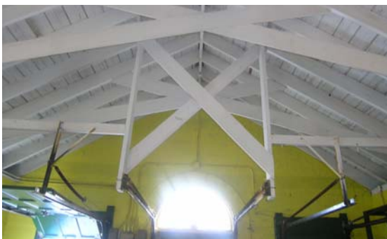
Roof Framing at Lobby
