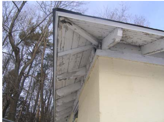
Eave Framing and Trim at southeast corner
