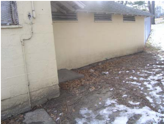
Walls at southwest corner.
