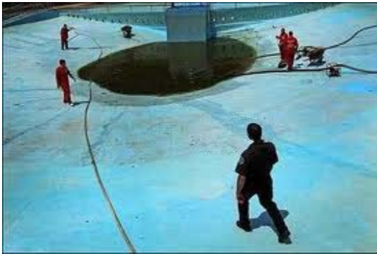
Routine Repairs in 2011
