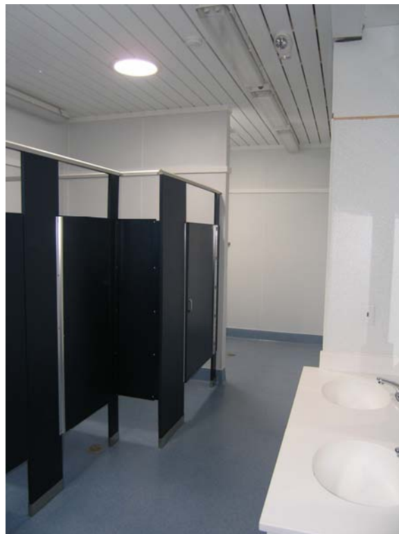
Example of FRP Walls, Epoxy Floor, Solid Plastic Partitions Slat Ceiling and Light /Tube
