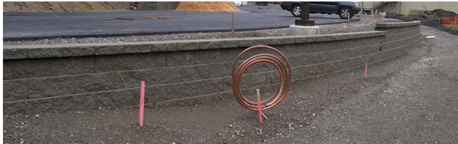
Example of Segmental Retaining Wall
