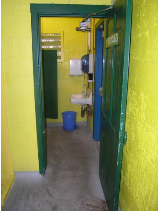
View into Men's Room
