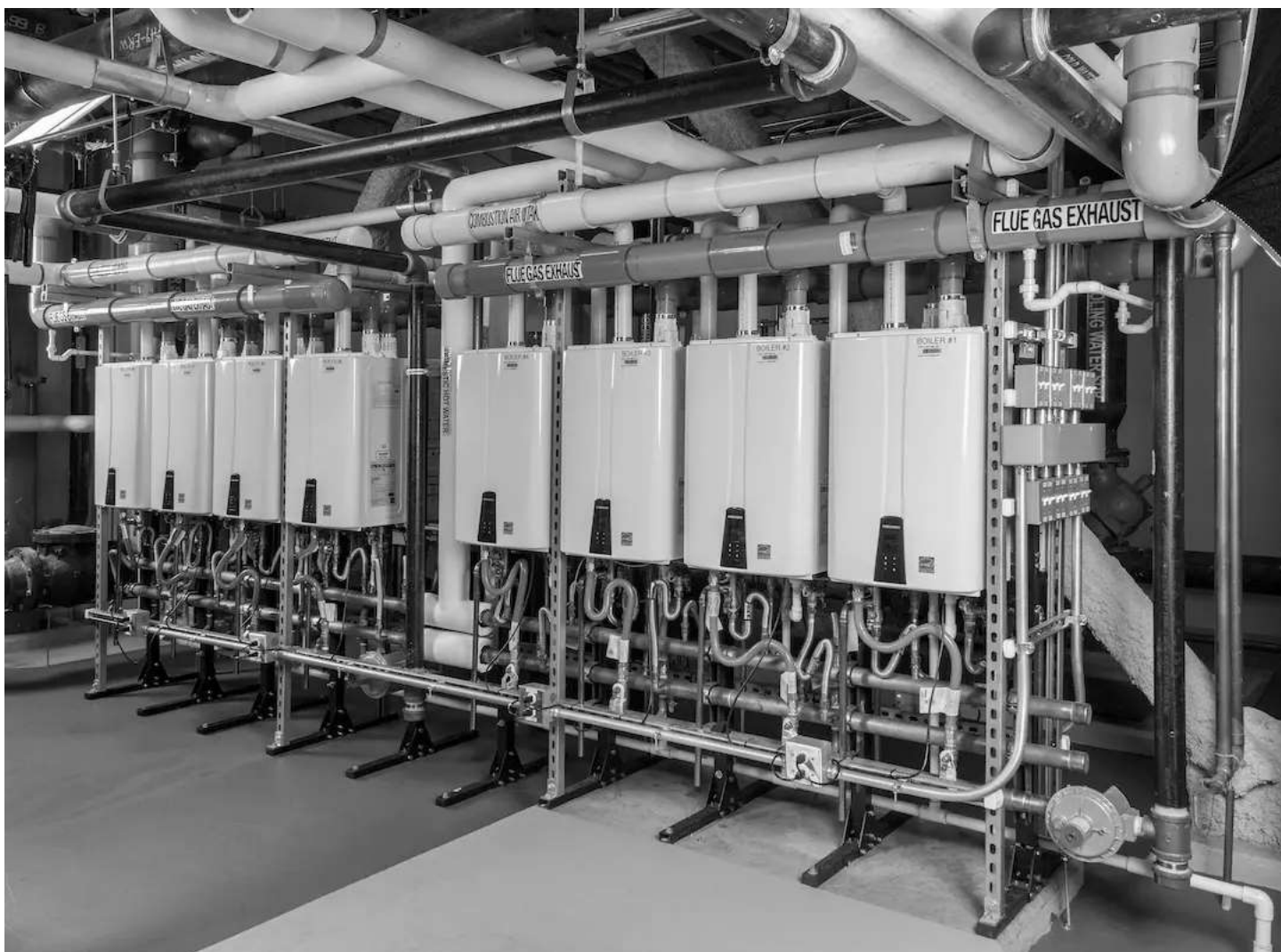
Navien NPE tankless water heaters "ganged" at West End Asteria Apartments, Boston. Photo: Navien Inc.
