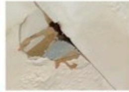
5. Ceiling with water damage in multiple areas
