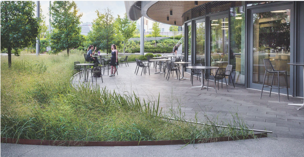
Rain Garden with corten steel edge, switch grass and blue flag iris
