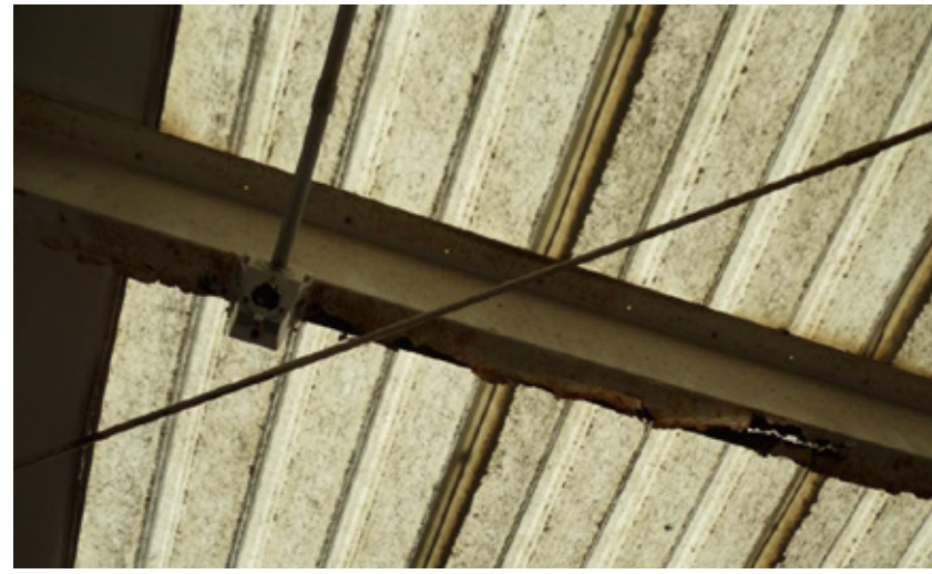
Rusted purlin with visible loss of section
