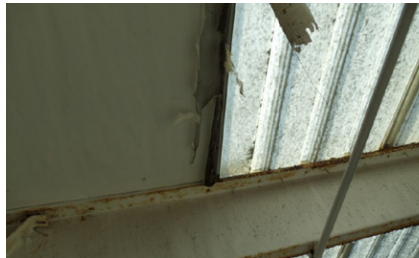
Deteriorated roof panel insulation
