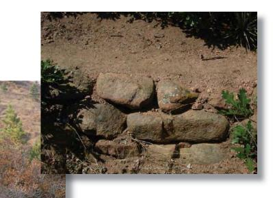
Stone retaining walls do not need to be complex. Simple walls provide great protection benefit to the trail surface and also provide easier and safer trail passage for trail users of all types.
