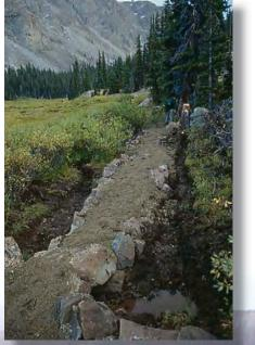
Natural resource impacts and safety issues resulted from poor original design where appropriate cross-trail drainage was included in the initial construction. A lesson learned: this rehabilitation project required more effort than the original implementation project. Initial placement of an appropriately designed armoring structure would have saved precious resources to address other areas of need.
