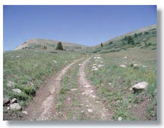
This two-track road in Colorado's high country, like most old 4-wheel drive roads, will not support sustainable trail use and therefore should not be considered for new trail design. It is too steep and crosses the prevailing cross slope at too great an angle. Erosion gullies have already started to form.
