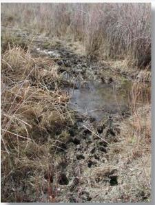
Even small swales that are not crossed properly or improved can deteriorate rapidly in muddy messes, causing natural resource, visual resource and water quality impacts. These impacts can be avoided by designing drainage improvements into the original new trail design.
