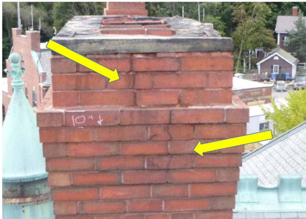
1. North Elevation. Fractures 10" from top
