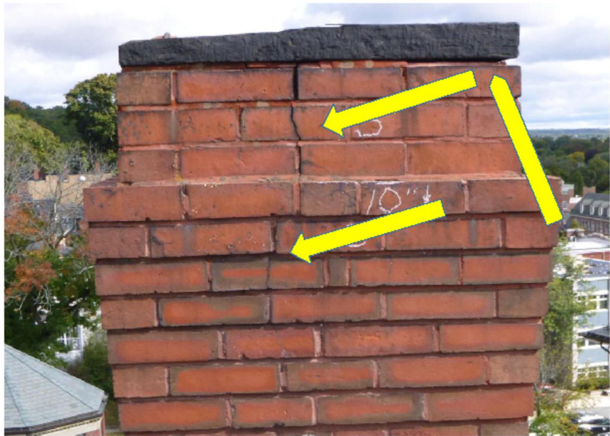
7. South Elevation. Fractures 10" from top
