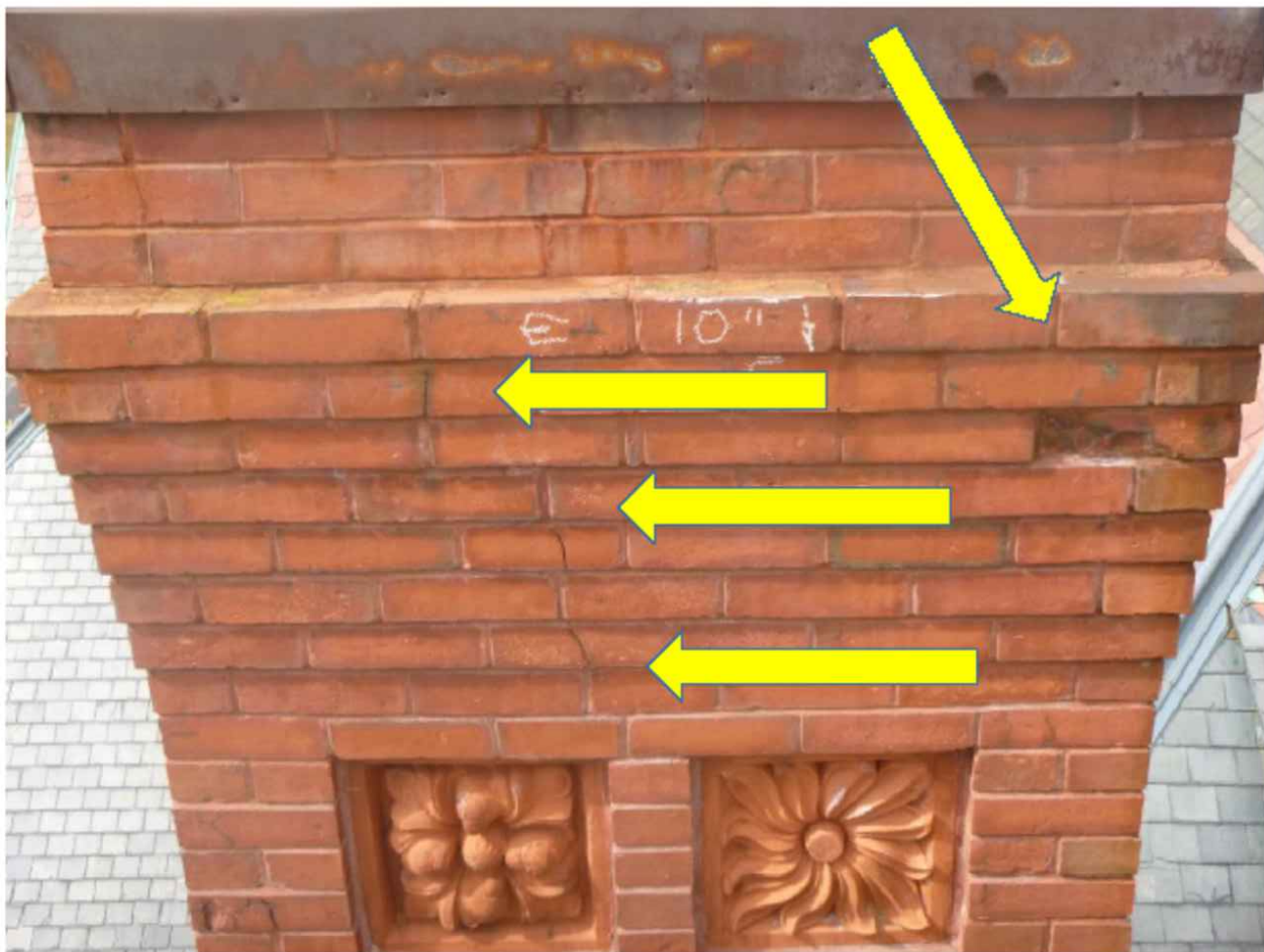
2. East Elevation. Fractured and Replace damaged brick & mortar
