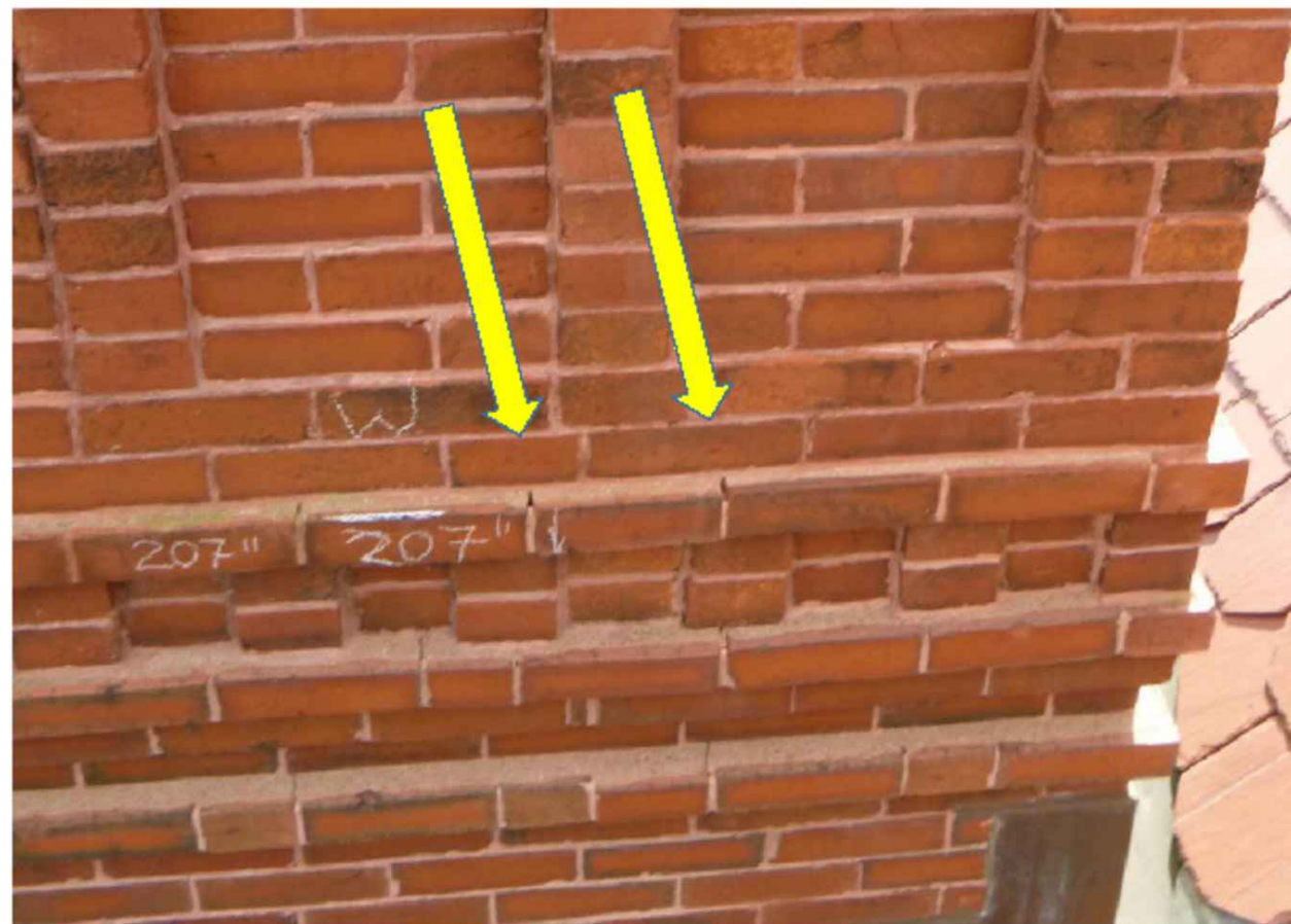
15. West Elevation. Open mortar joints at 207" from top
