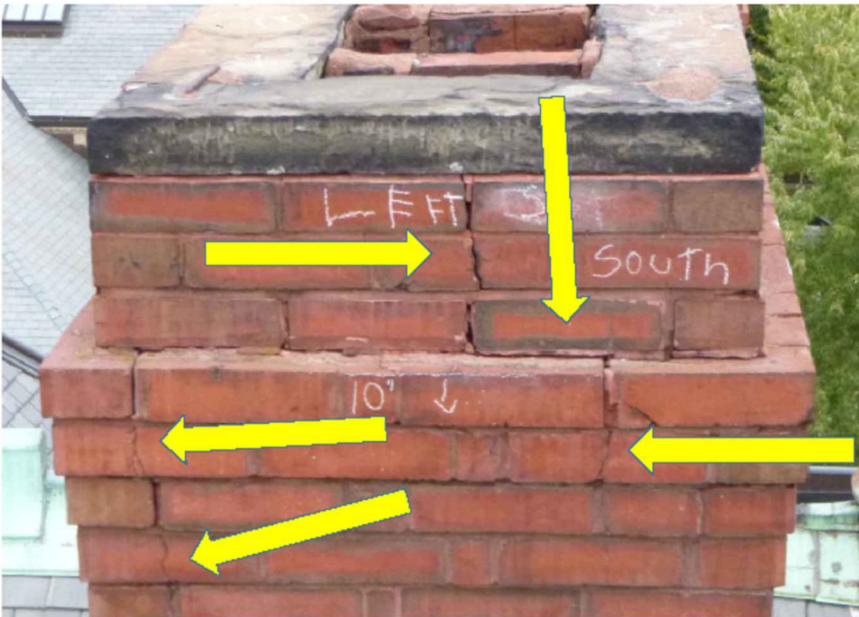
6. South Elevation. Fractures and Repoint open mortar joints 10" from top
