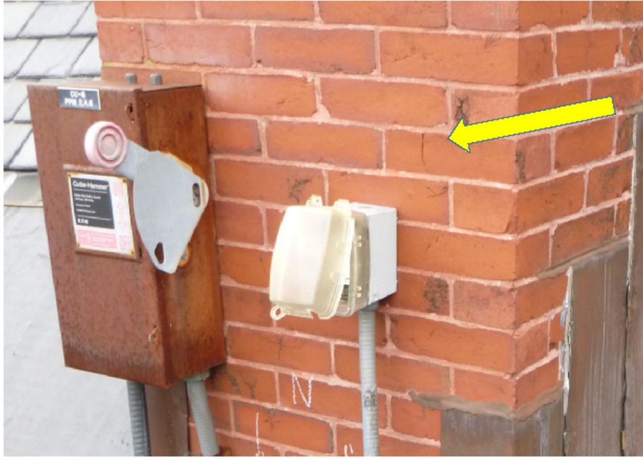
3. North Elevation. Fractures 255" from top
