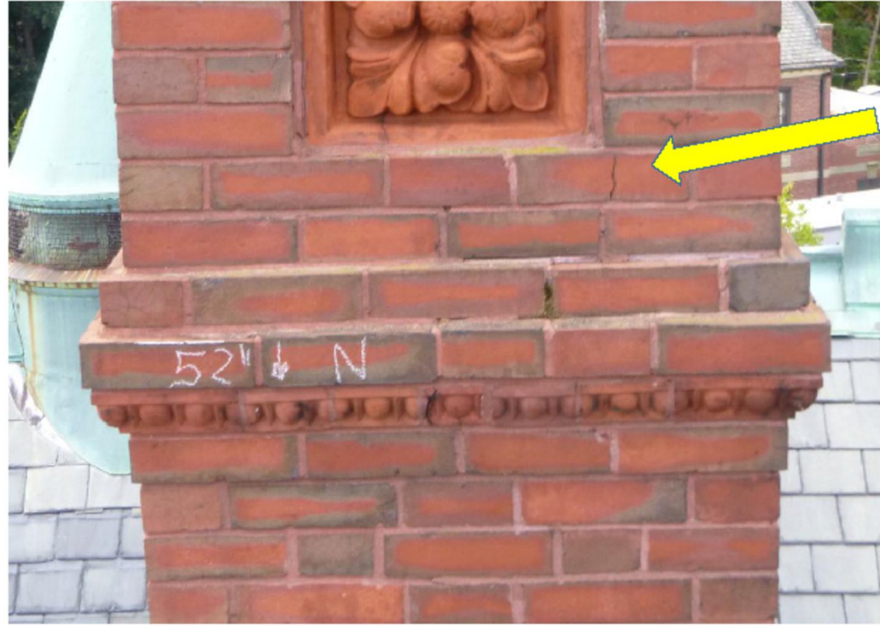
2. North Elevation. Fractures 48" from top
