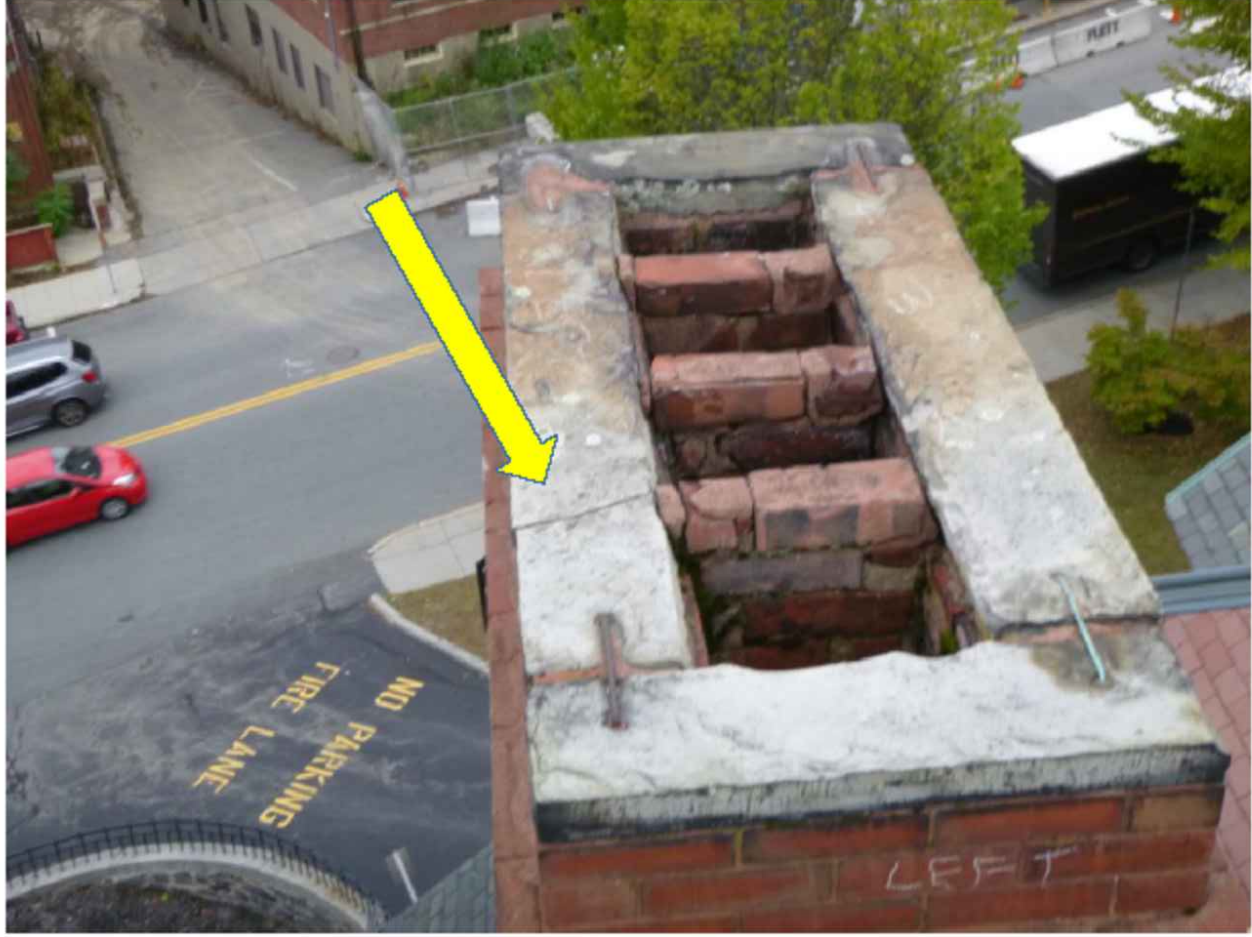
1. Fracture in Cap
