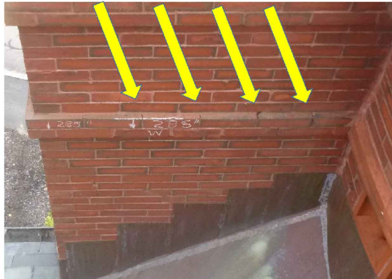
7. West Elevation. Repoint open mortar joints 285" from top
