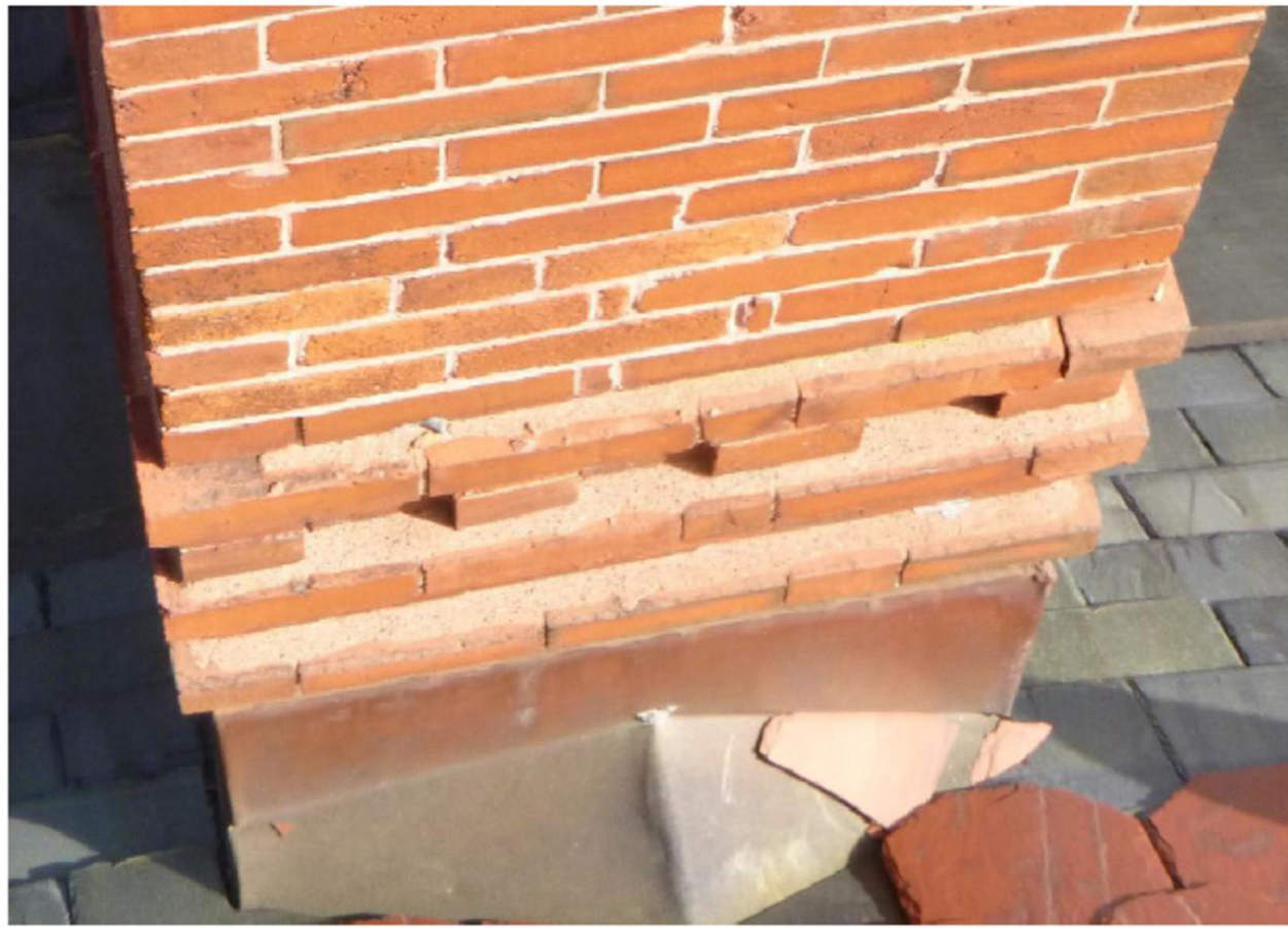
10. South Elevation. Open mortar at base of chimney
