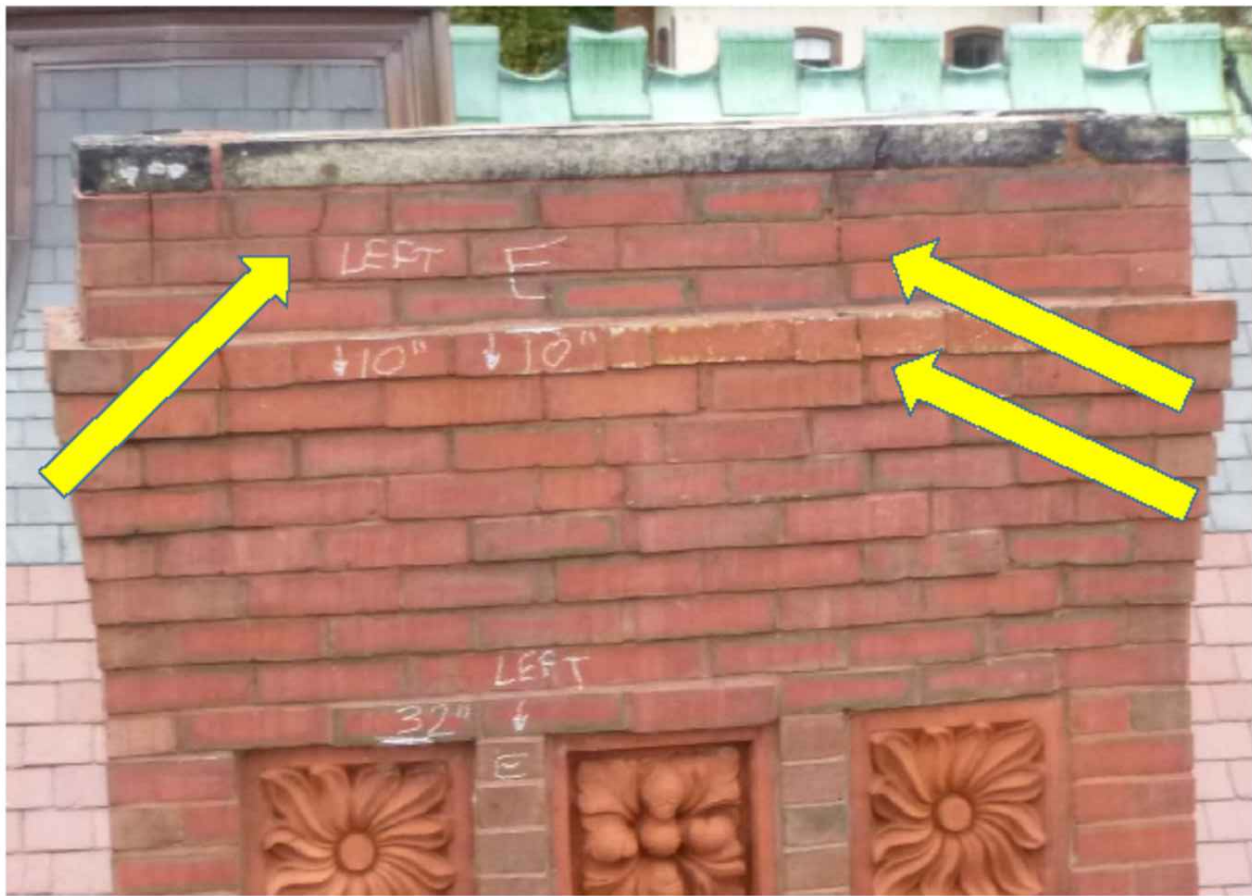
4. East Elevation. Replace fractured brick &
