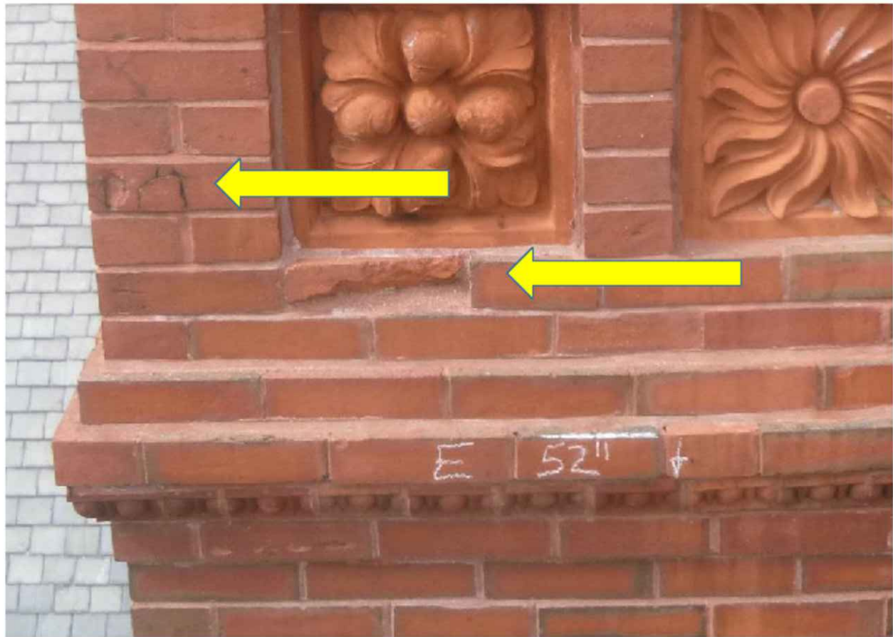
3. East Elevation. Replace damaged brick & mortar 48" from top.
