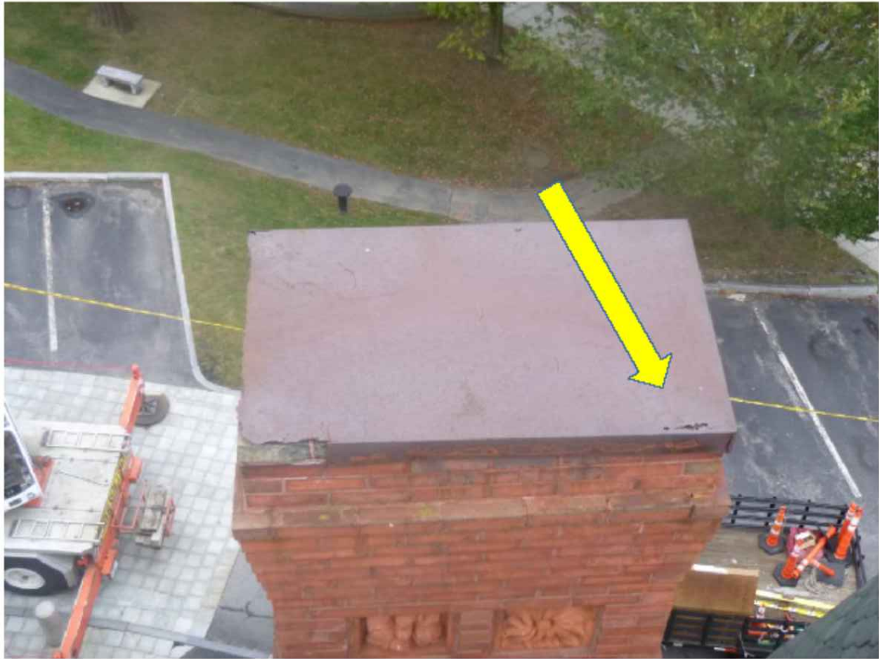
1. Deteriorated Chimney Cap
