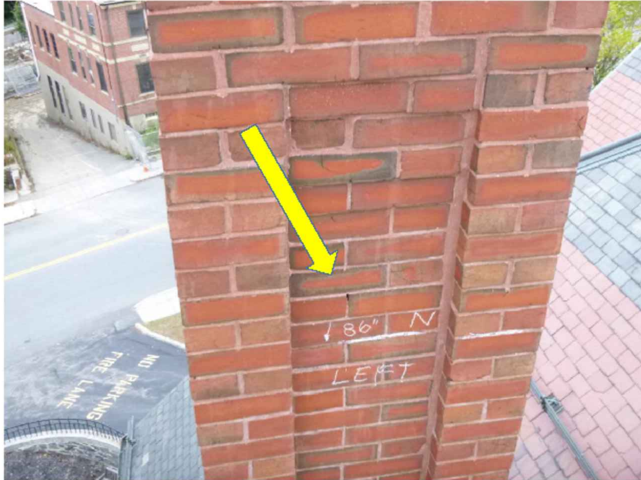
2. North Elevation. Open mortar joint
