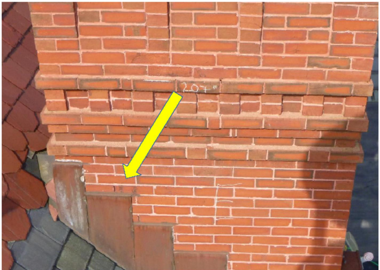
6. East Elevation. Repoint open mortar joints 228" from top
