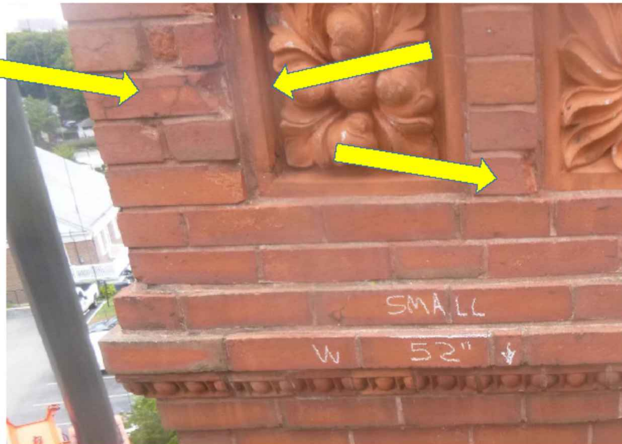
6. West Elevation. Replace damaged brick & mortar 40" from top.
