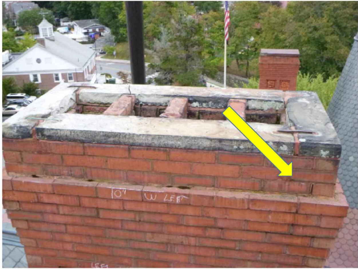
8. West Elevation. Open mortar joint 10" from top
