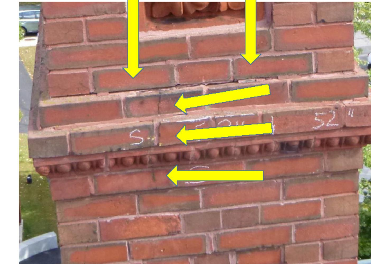
8. South Elevation. Deteriorated mortar joints 50" from top
