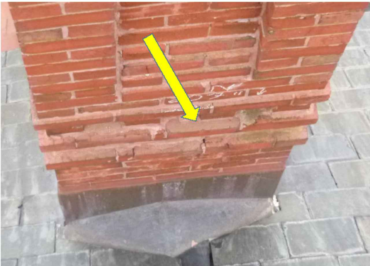
3. North Elevation. Open mortar joint at base of chimney
