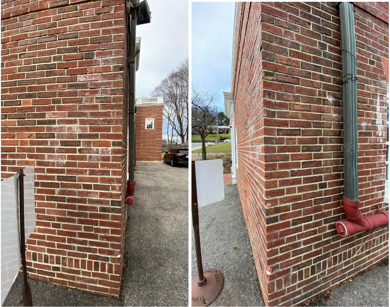
DAMAGED BRICKS AT CORNER OF FAÇADES 11 AND 1. REPLACE BRICKS, REPAIR AND POINT MASONRY.
