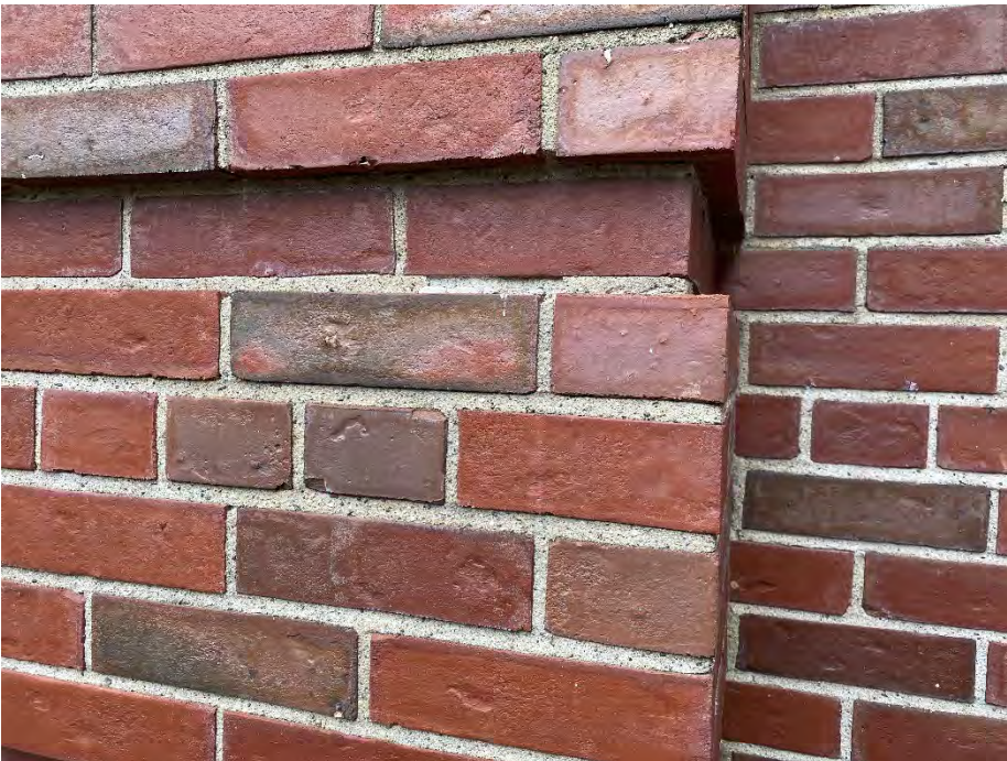
PILASTER MORTAR NEEDS POINTING
