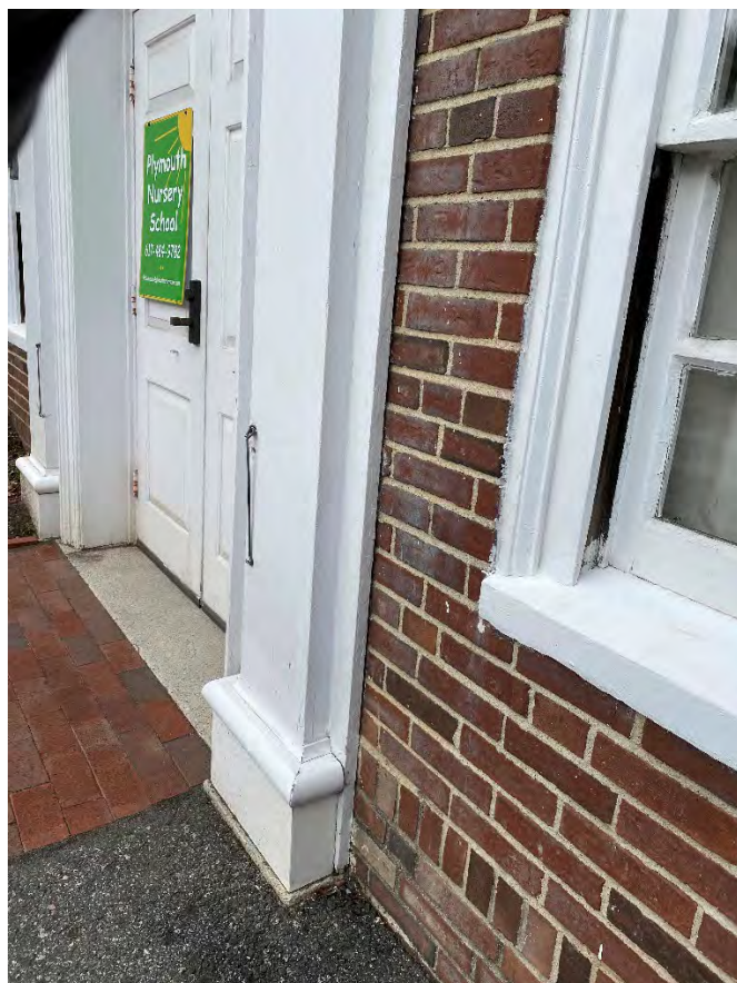
INSTALL SEALANT AT WOOD/MASONRY JOINT AT FRONT DOOR
