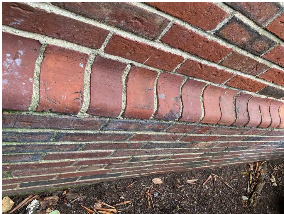
WATERTABLE REQUIRING POINTING A
