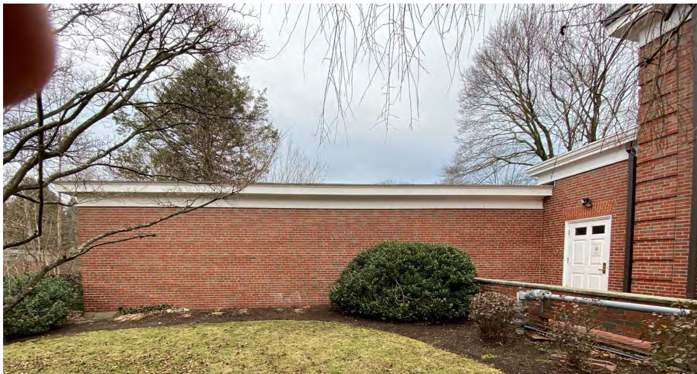
OVERALL VIEW OF FAÇADE 5. BRICKWORK GENERALLY IN GOOD CONDITION
