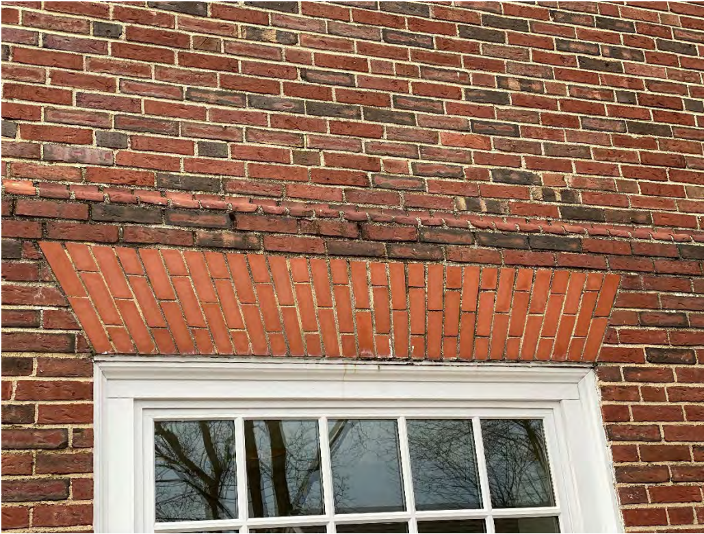
DETAIL OF WATERTABLE NEEDING POINTING
