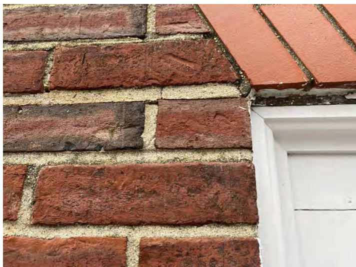
GENERALLY POINT MASONRY, AND REPLACE SEALANTS AT LINTELS
