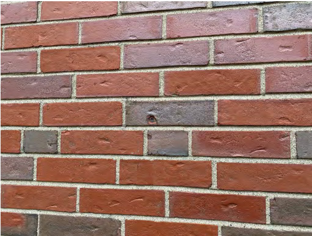
METAL OBJECT(S) IN BRICK(S) NEED REMOVAL AND/OR PATCHING.
