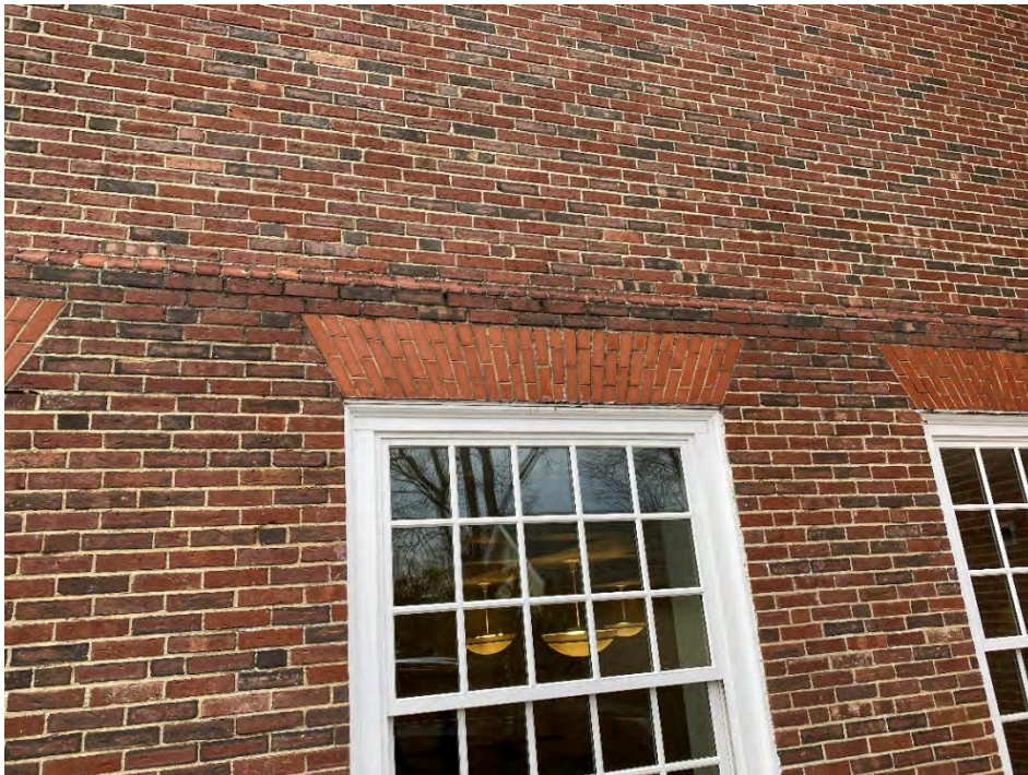
CLOSE-UP OF DETERIORATED WATERTABLE LEDGE
