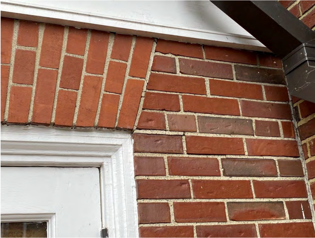
DETAIL AT DOOR WITH LOOSE MORTAR AND POINTING REQUIRED A
