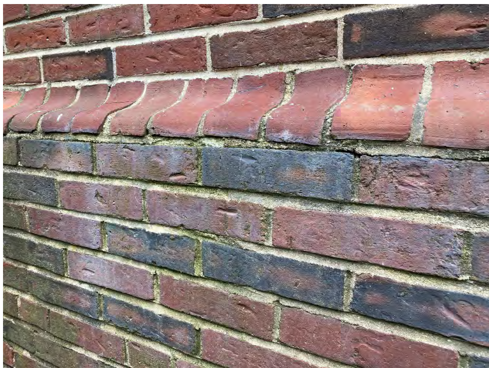
WATERTABLE REQUIRING POINTING B
