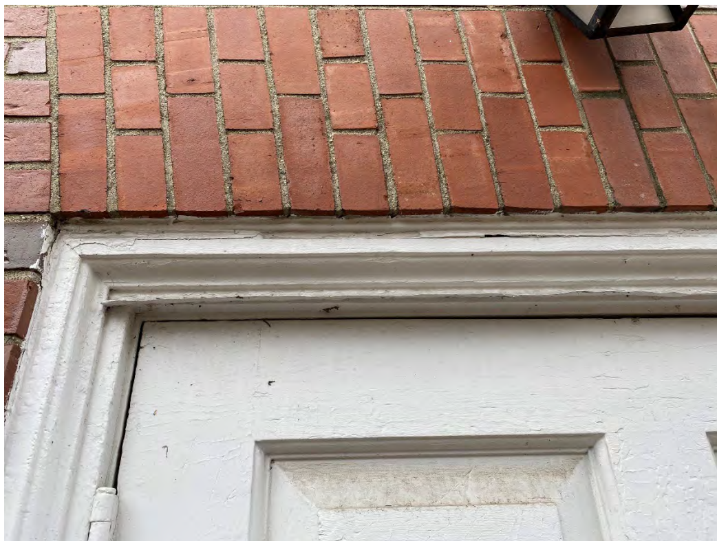
SEALANT REQUIRES REPLACING AT DOOR ON FAÇADE 3
