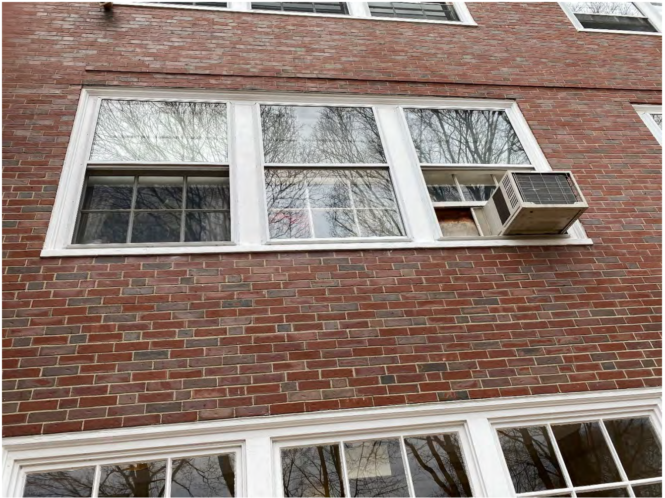
PARTIAL FAÇADE 2. LINTEL AT SECOND FLOOR REQUIRES SEALANT.
