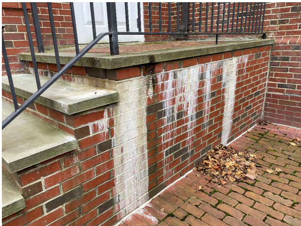
DETAIL OF FACE OF STAIR AND PLATFORM WITH LEACHED SALTS TO BE CLEANED.
