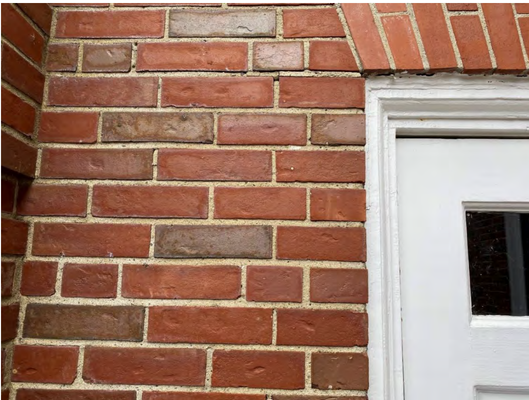
DETAIL AT DOOR WITH LOOSE MORTAR AND POINTING REQUIRED B
