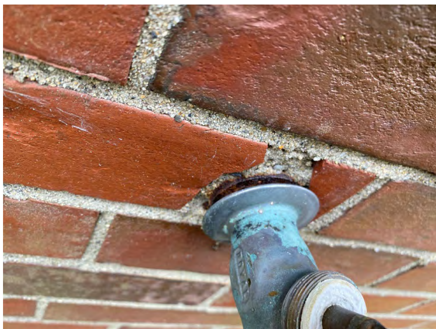
HOSE BIB PENETRATION REQUIRES SEALANT
