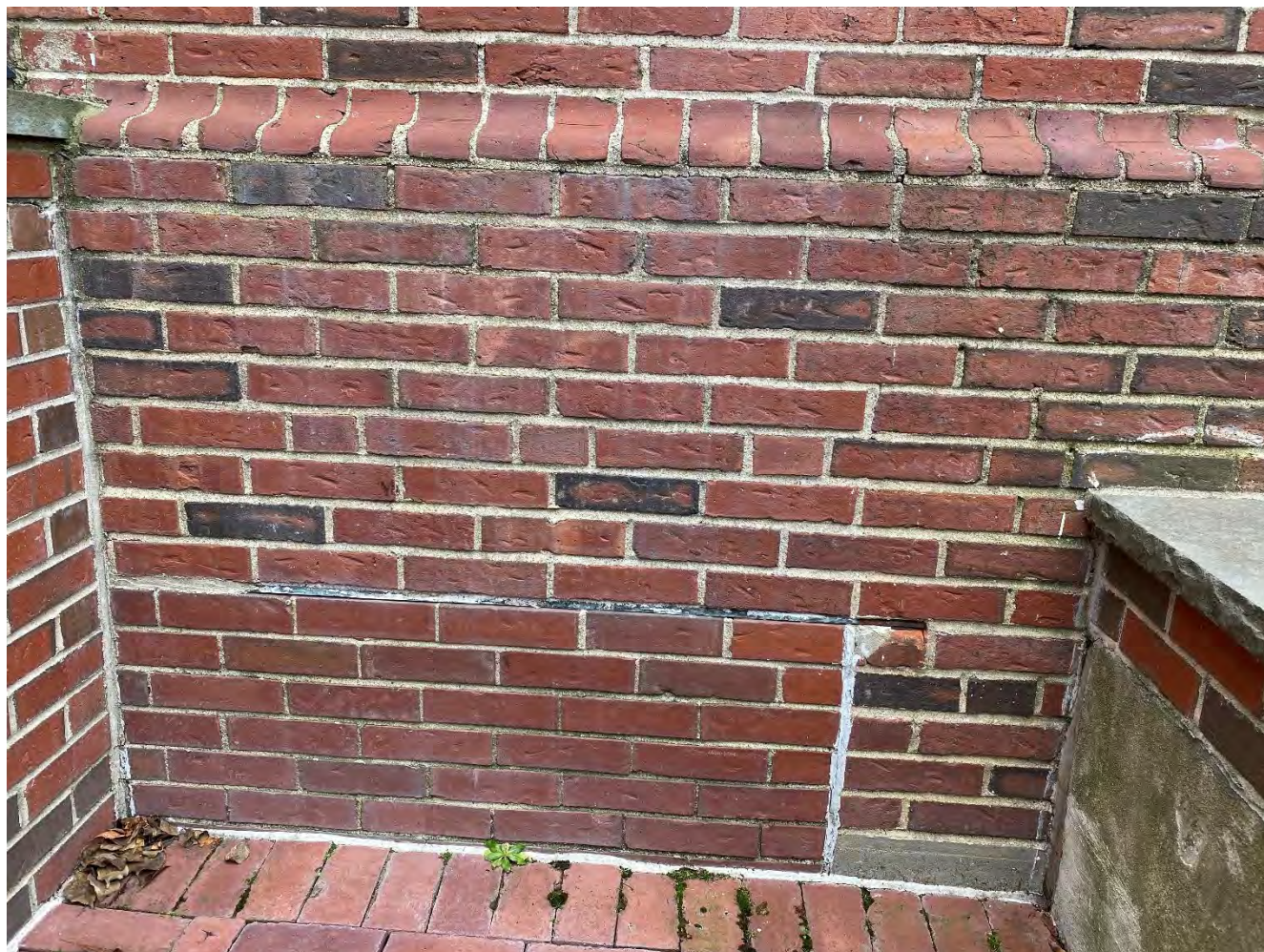
WATERTABLE BRICK REQUIRES POINTING. EXPOSED LINTEL REQUIRES SEALANT. DAMAGED BRICK REQUIRES REPAIR.
