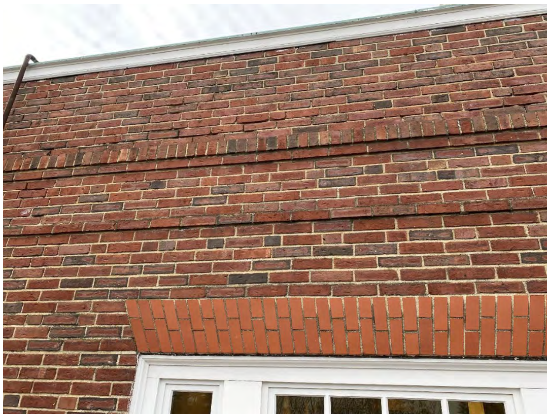
FAÇADE 1 CLOSE-UP OF MASONRY BANDS REQUIRING POINTING ALONG WHOLE LENGTH OF FAÇADE.
