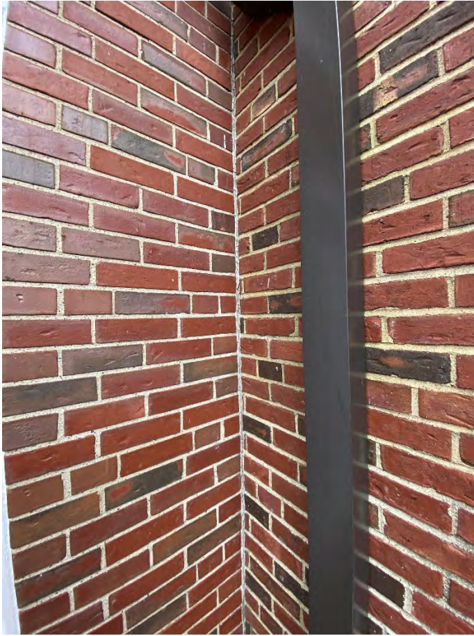
CORNER JOINT NEEDS NEW SEALANT
