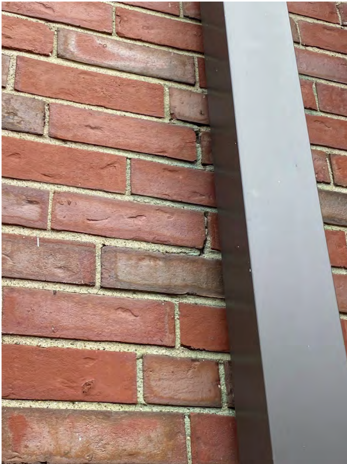
NEXT TO LEFT DOOR: MORTAR LOOSE, MISSING. NEEDS POINTING.
