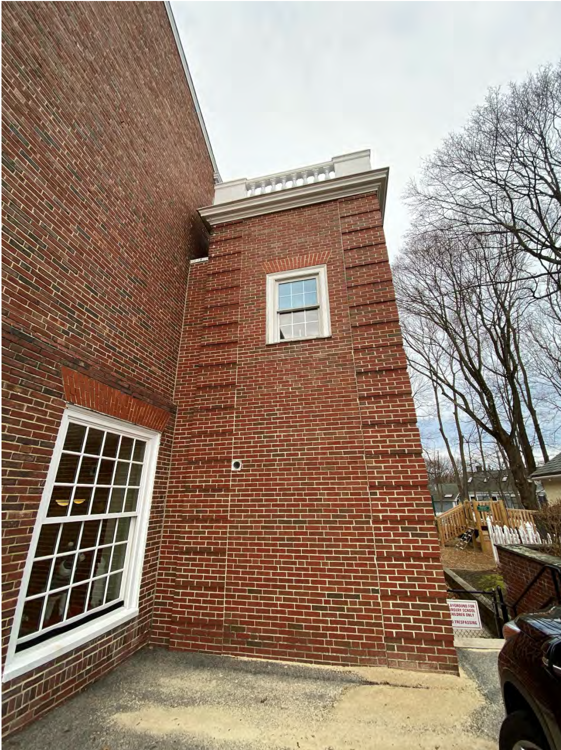
ELEVATOR SHAFT ADDITION MASONRY IN GOOD CONDITION. RIGHT (EAST) END OF FAÇADE 1.
