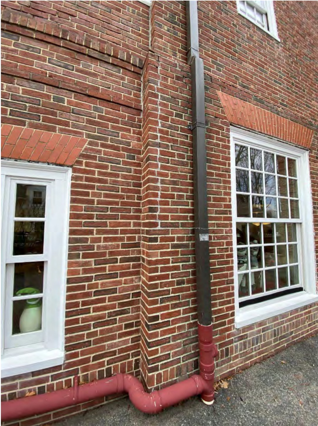
JOINT BETWEEN HIGH & LOW PORTIONS WITH CRACKED MASONRY NEAR CORNER. REQUIRES BRICK REPLACEMENT, POINTING, AND SEALANT REPLACEMENT.
