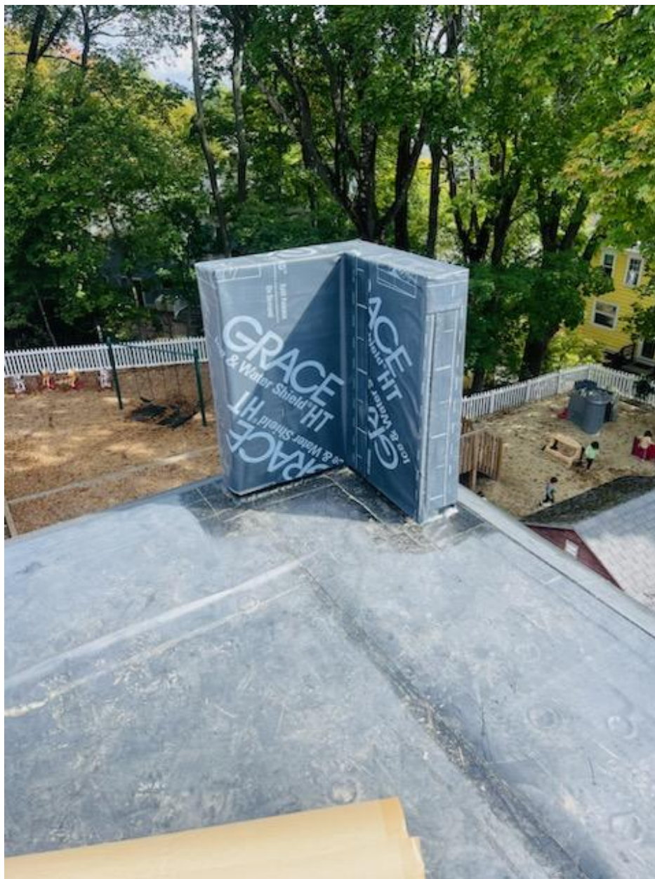
One of four water proofed corner structures
