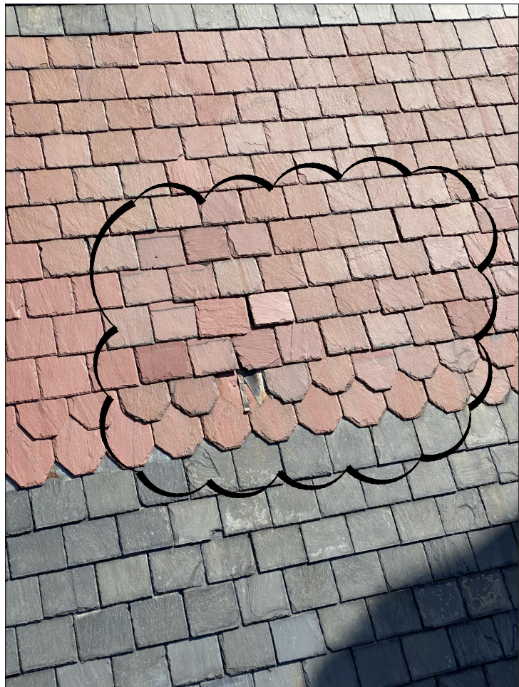
7. Typical damaged and Missing Slate
