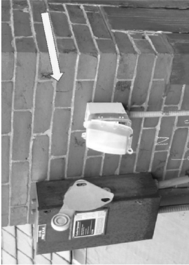
3. North Elevation. Fractures 255" from top
