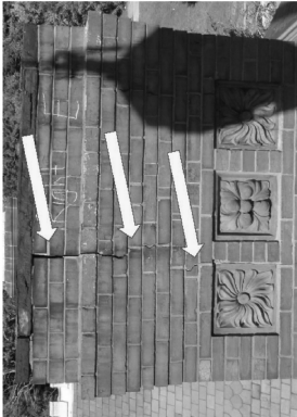
4. East Elevation. Fractures & open mortar joints 10" from top
