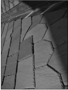
8. Damaged Slate & Mismatched Color
