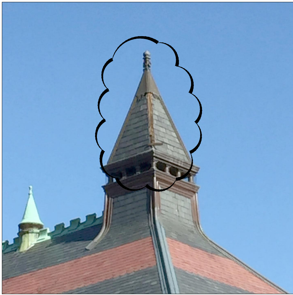
2. Damaged Hip on South Spire
