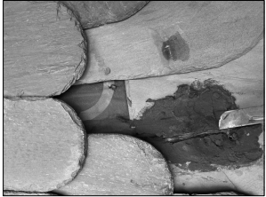
3. Damaged & missing Slate
