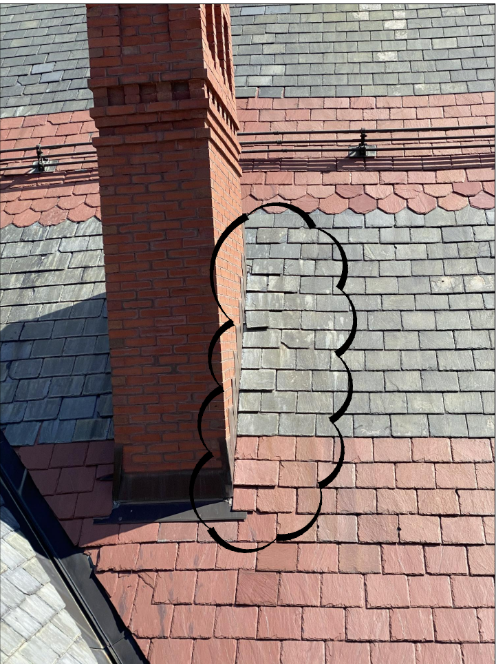
6. Typical Damaged Slate
