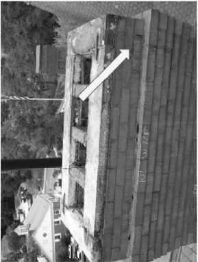
8. West Elevation. Open mortar joint 10" from top
