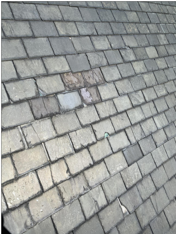
5. Damaged, cracked and broken Slate
