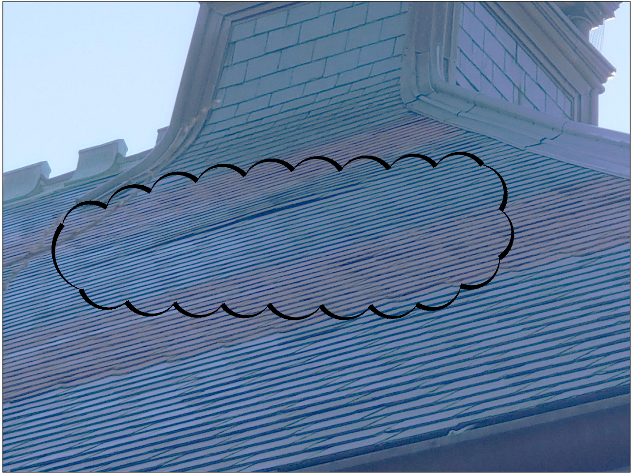
1. Raised Slate. Sheathing Damaged
