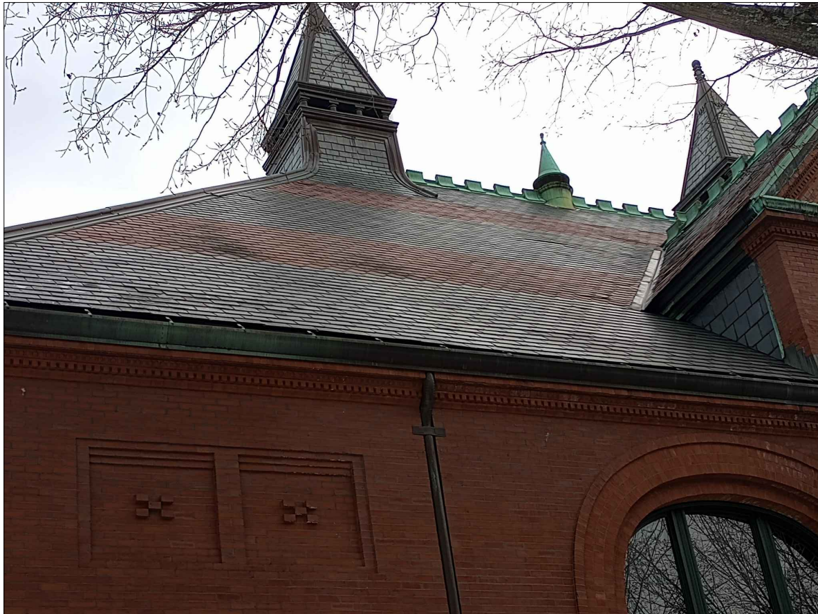
10. Raised Slate. Sheathing Damaged
