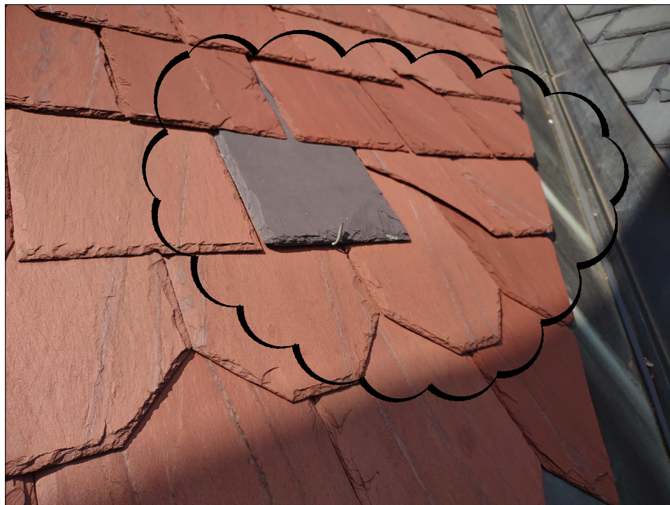
8. Damaged Slate & Mismatched Color
