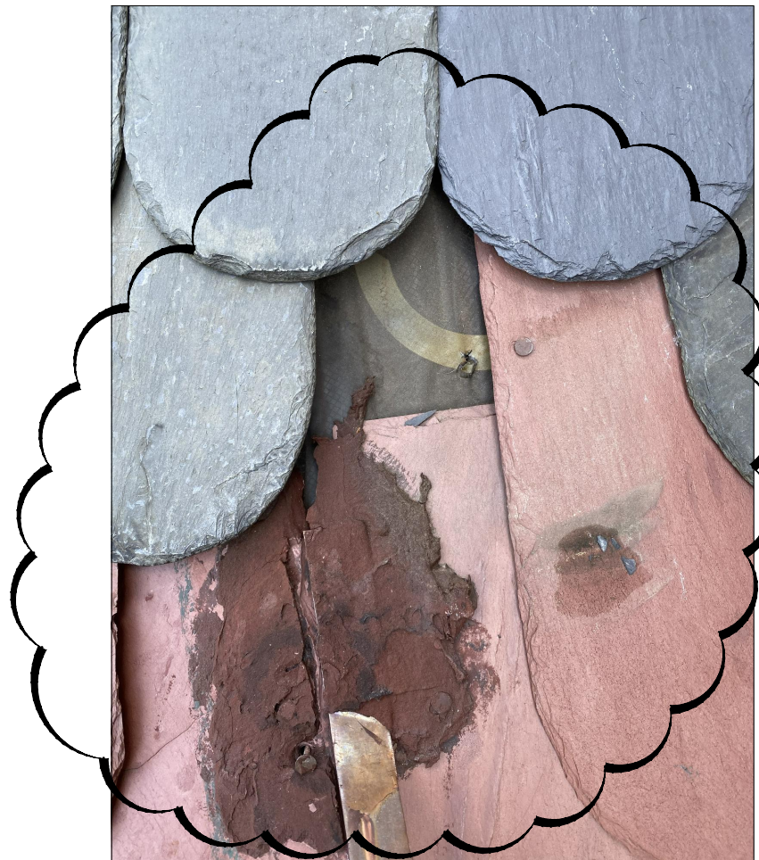
3. Damaged & missing Slate
