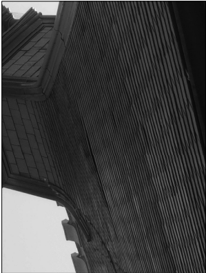
1. Raised Slate, Sheathing Damaged
