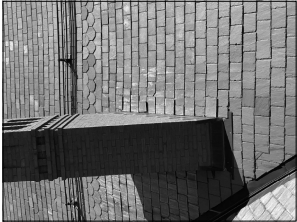
6. Typical Damaged Slate
