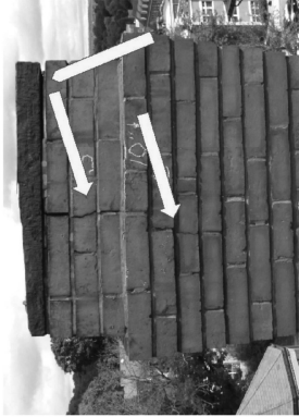
7. South Elevation. Fractures 10" from top
