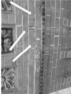
5. East Elevation. Open mortar joints 52" from top
