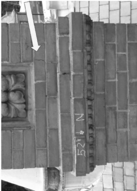
2. North Elevation. Fractures 48" from top
