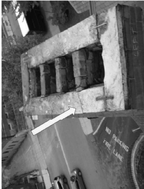
1. Fracture in Cap
