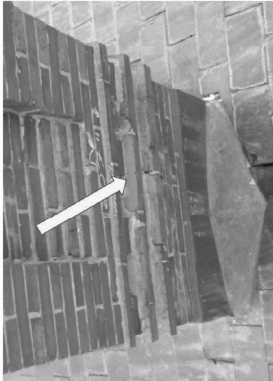
3. North Elevation. Open mortar joint at base of chimney
