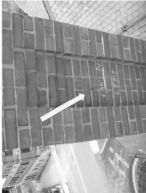
2. North Elevation. Open mortar joint
