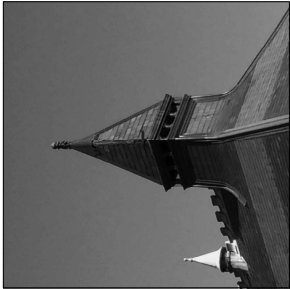
2. Damaged Ridge on South Spire
