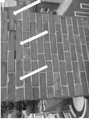
9. South Elevation. Horizontal fractures 100" from top
