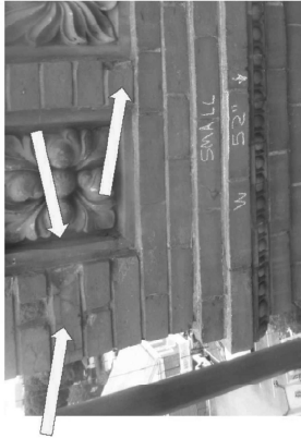
6. West Elevation. Damaged brick 40" from top.
