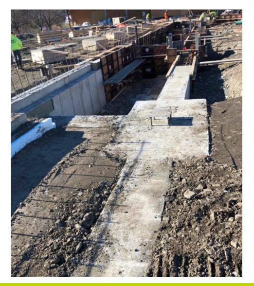
Area D Grade Beam and Pile Cap Concrete and Formwork
